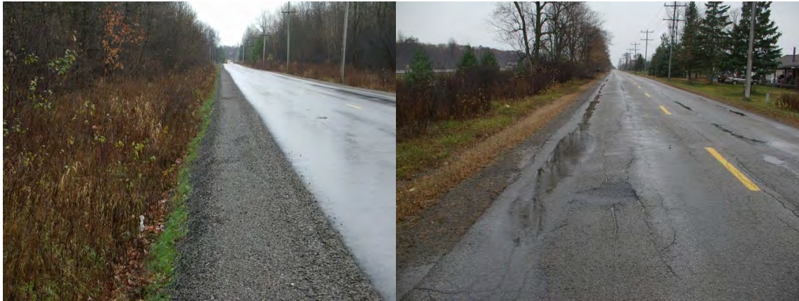
Figure 12 Steep Side Slopes
