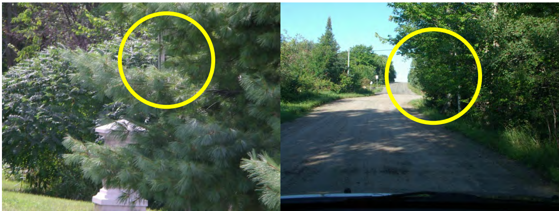
Figure 19 – Obscured Regulatory Signage
