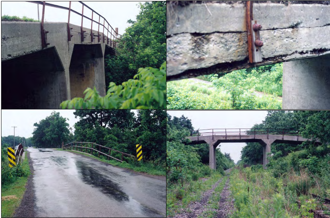
Figure 5 'NOW' Need Bridge
