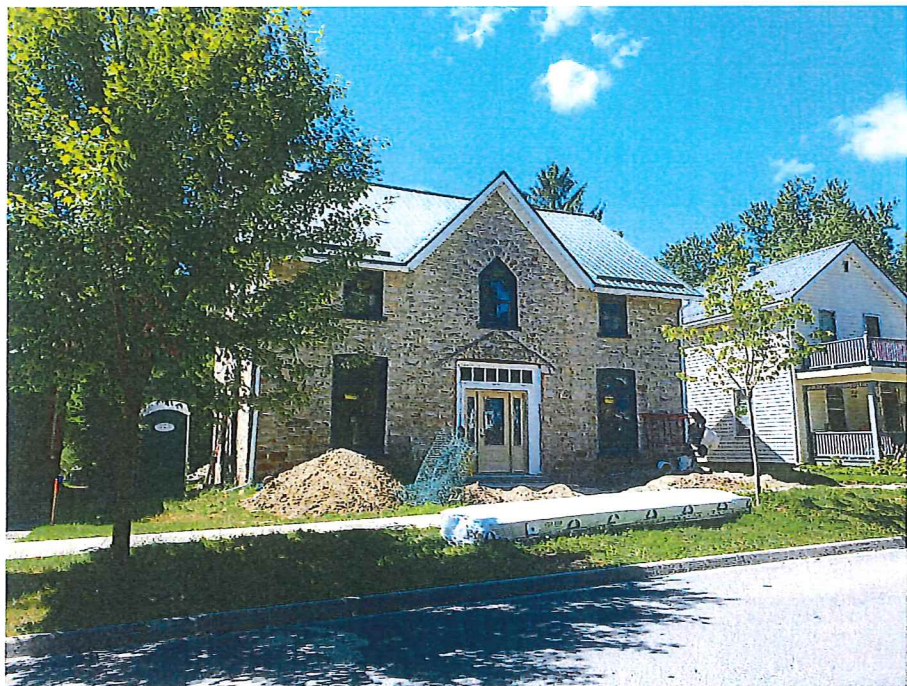
Figure 3 & 4 – Front view of subject property, 40 Princess Street.
