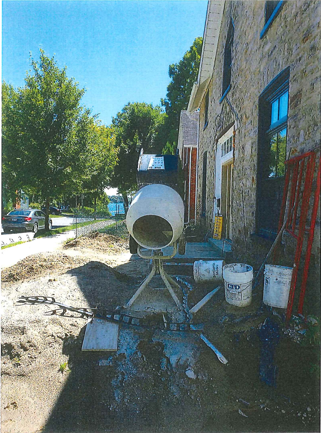
Figure 7 – View of subject property, facing South
