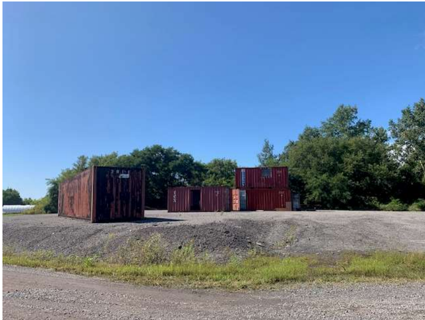
Location of the new fire training facility looking west
