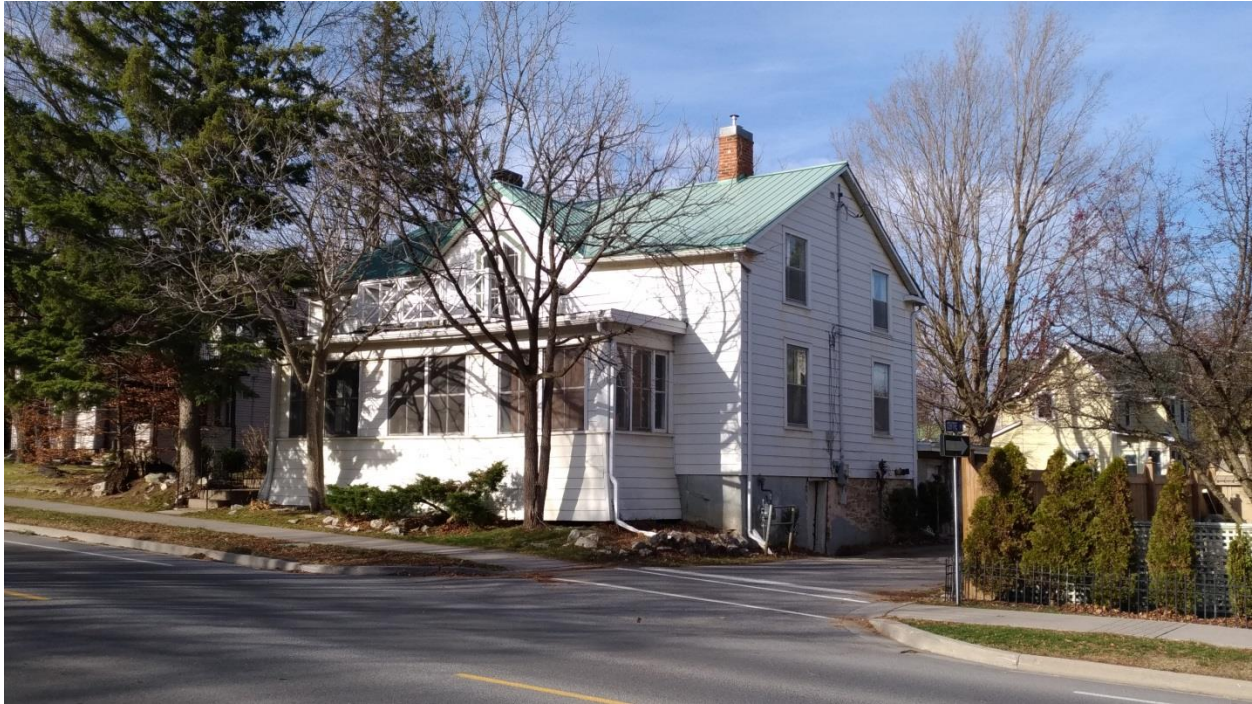
Figure 1: 120 King Street West, viewed from the southeast (E. Tumak, Nov. 2020).
