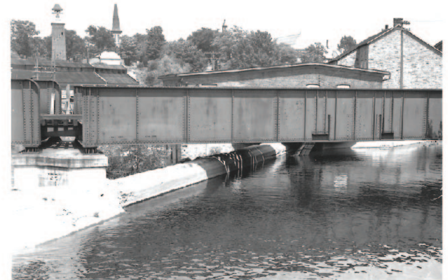
Pictured here in a 1956 photograph, is the trestle connecting King and Mills Streets. The lower dam was once situated below the trestle. That dam was removed in 1991.
