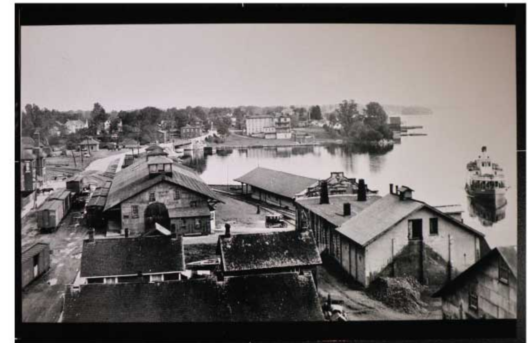
The Gananoque Swing Bridge connects Water Street on the west to the intersection of John and Stone Street.
