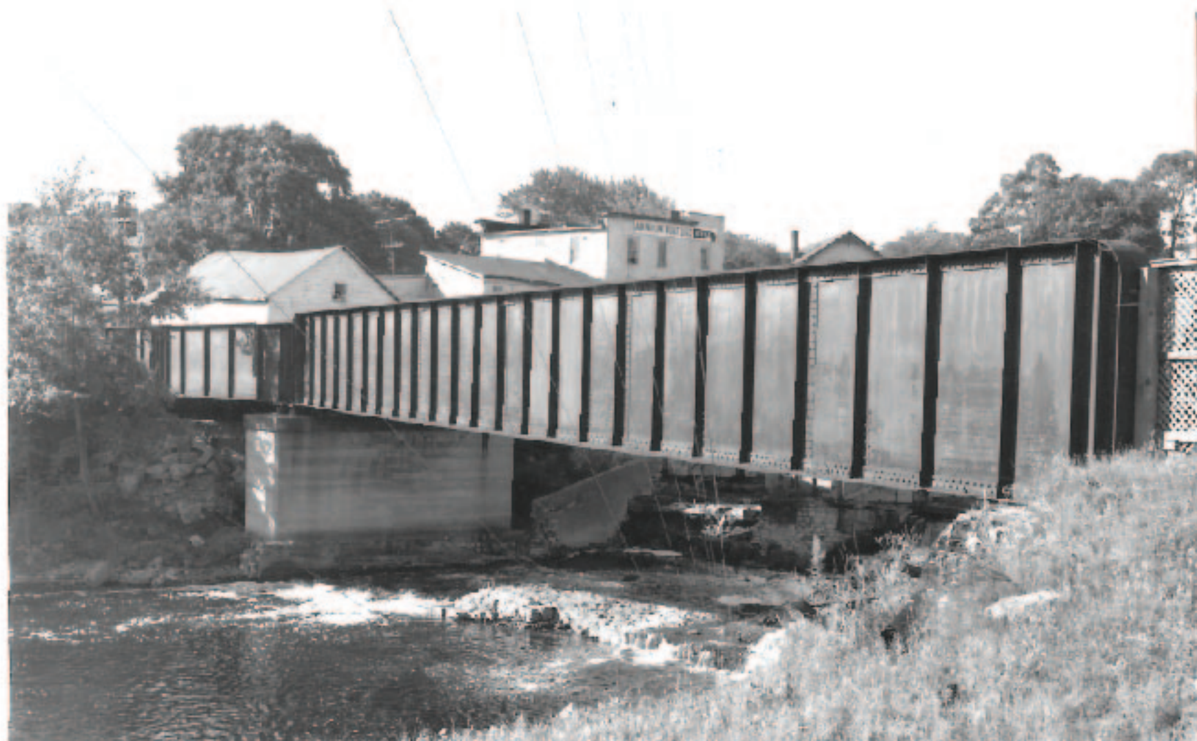
The trestle that connects King and Mill Street (above, in 1956) is one of two remaining trestles of the Thousand Island Railway that cross the Gananoque River.
