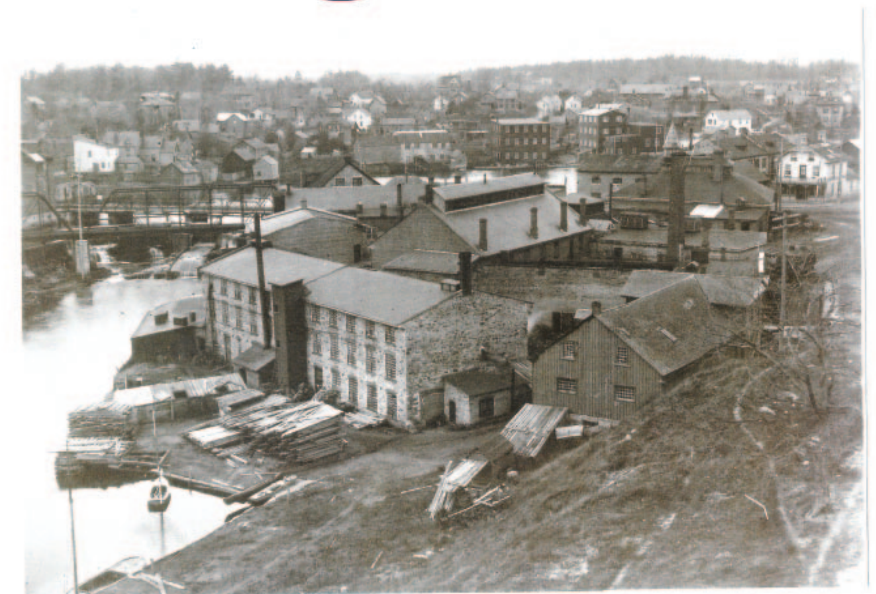
The original trestle, built in 1884, can be seen in this aerial photo of Lower Gananoque. The trestle provided part of a vital link to the Grand Trunk Railway for Gananoque's many manufacturers.
