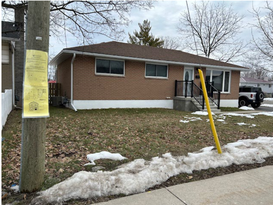
View of the front of the existing dwelling at 95 Elizabeth Drive
