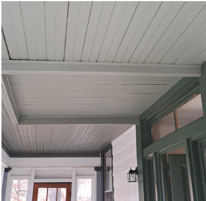
Figure 4. Front porch of 120 King St. West showing portico aperture and presumed original ceiling
