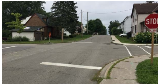
Figure 5: Intersection of William Street N and North Street, Looking South
