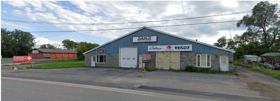
The front of the vacant building where the proposed manufacturing facility will operate
