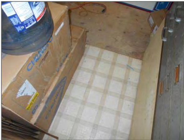
Non-asbestos vinyl sheet flooring present in the basement furnace room.
