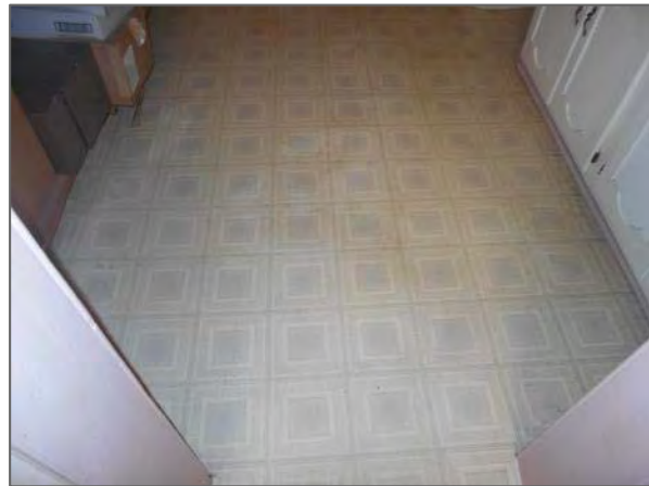
Non-asbestos vinyl sheet flooring present in the basement women's washroom.
