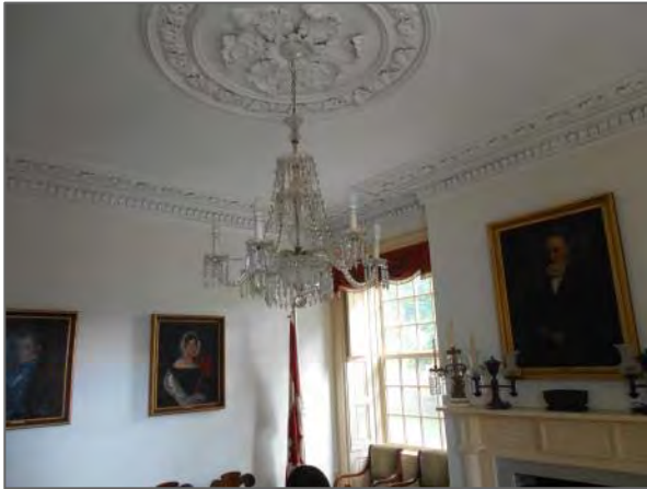
Non-asbestos plaster present throughout the building.
