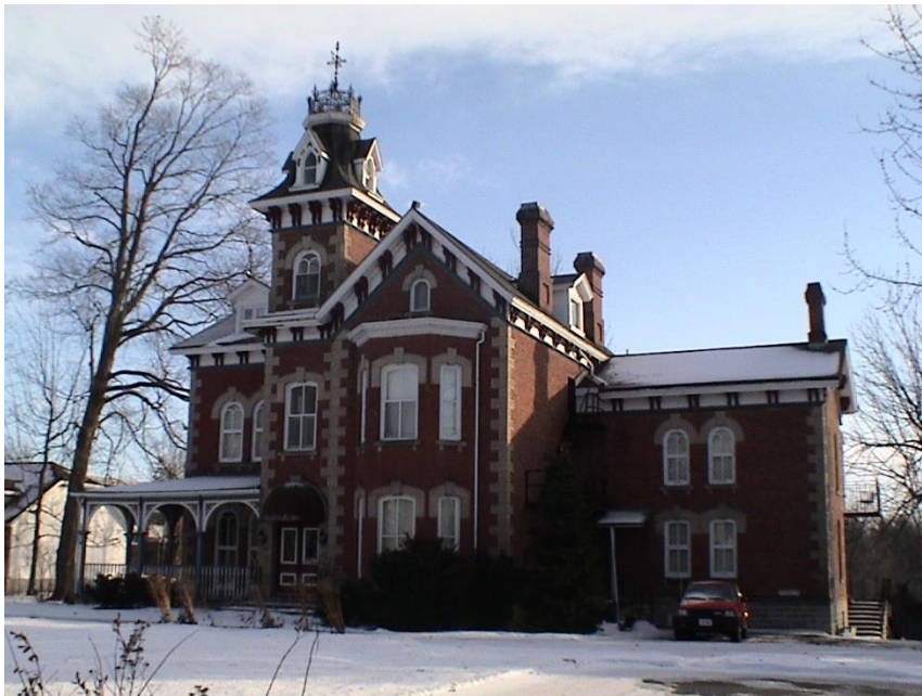
Figure 18: 279 King Street West, viewed from the northwest, former Samuel McCammon residence, 1872, in the Italian Villa style (photo E. Tumak, Jan., 2008).
