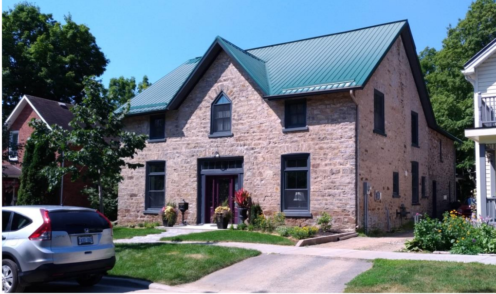
Figure 8: 40 Princess St., the first Christ Church Rectory, viewed from the northeast, built after the first phase of Christ Church 1857-58, enlarged at the rear late 1910s. It is an example of what is often called an Ontario cottage form with embellishments in the Regency style (1830-60) for the door surround and a triangular topped central upper window in a Gothic Revival style mode in keeping with most of the windows of the associated Christ Church (photo E. Tumak, July 2009).
