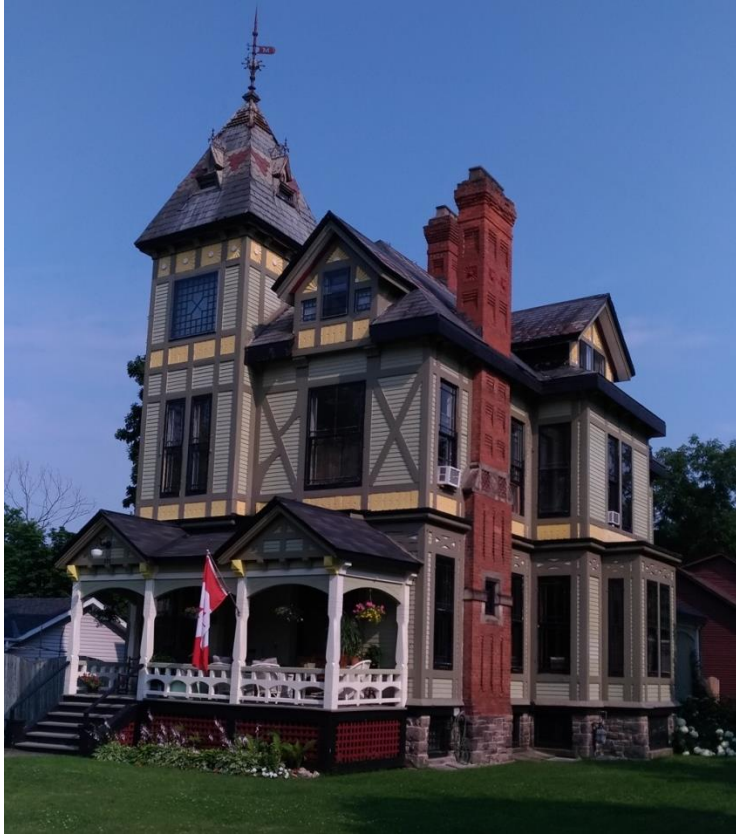
Figure 17: 375 King Street West, Brockville, viewed from the northwest (E. Tumak, July 2021).
