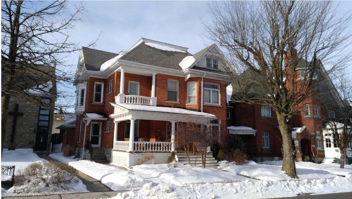
Figure 8: 128 Pine Street, viewed from the southwest with Grace United Church to the left and 136-38 Pine Street to the right (E. Tumak, Feb. 2020).
