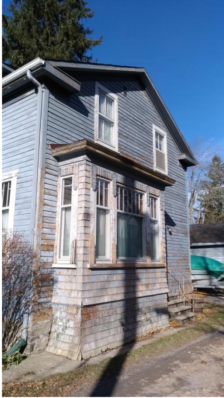
Figure 15: 145 Stone Street South, Gananoque, rear/original portion of ca. 1830 with 1884-85 bay window addition, viewed from the southwest facing Spruce Alley (E. Tumak, Nov. 2020).
