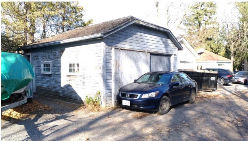
Figure 16: 145 Stone Street South, Gananoque, garage at east/rear end of property fronting onto Spruce Alley (E. Tumak, Nov. 2020).
