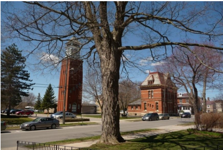
Figure 23: View to west side of Stone Street South, opposite the Dumble House and St. Andrew's Presbyterian Church, showing the Clock Tower on the left and the former Post Office on the right (E. Tumak, May 2015).
