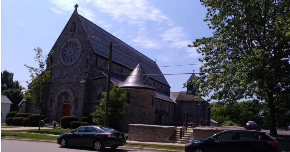
Figure 24: St. John's, viewed from the northeast with the former baptistry on the right foreground and the bell 'tower' and belfry on the right background (E. Tumak, July 2019).
