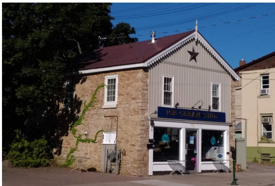
72 Stone Street South, viewed from the southeast (E. Tumak, Aug. 2019).
