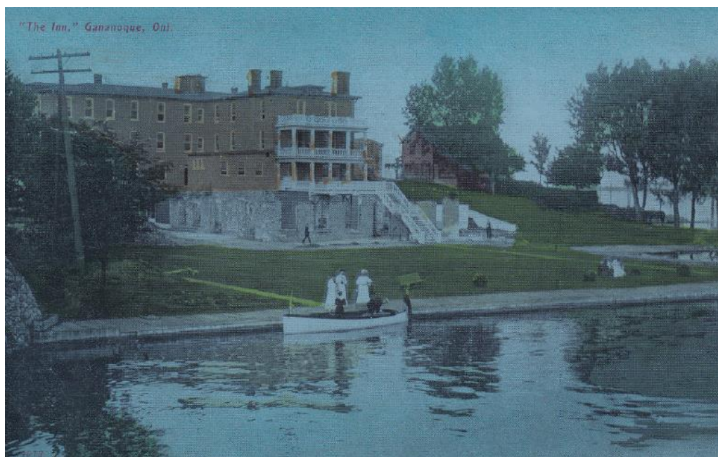
Gananoque Inn, viewed from the northwest, ca. 1910, showing the post-1907 fire rehabilitation (D. Rombough postcard and photographic collection).
