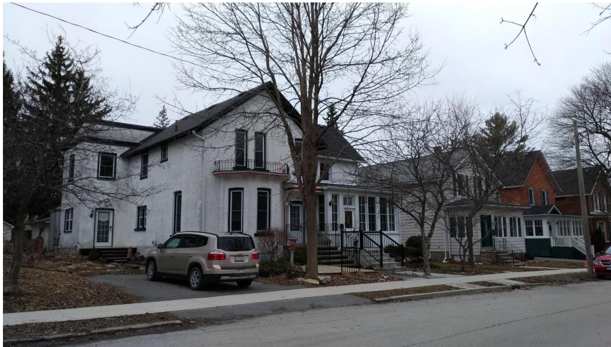
150-52 Sydenham Street, Gananoque, viewed from the southwest, former Convent of the Sisters of Providence (E. Tumak, Sept. 2019).
