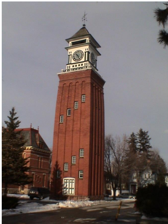
140 Stone Street South, Gananoque Clock Tower, viewed from the southeast (E. Tumak, Jan., 2008).
