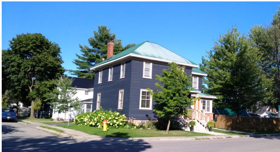
93 William Street North, viewed from the northwest (E. Tumak, Aug. 2019).
