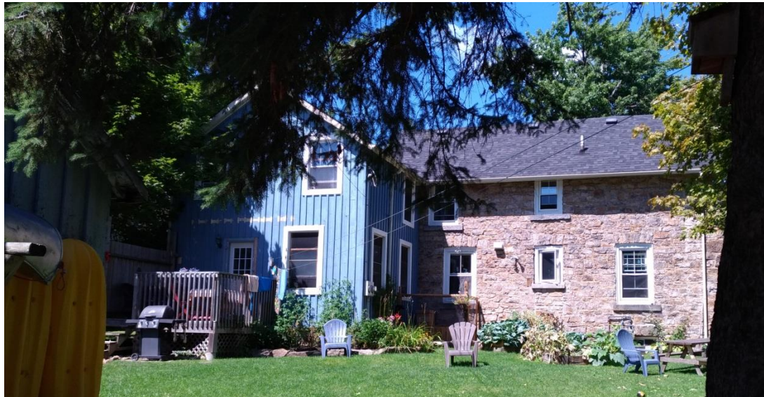
153 Sydenham Street, rear elevation viewed from Cedar Alley from the southeast (E. Tumak, Aug. 2019).
