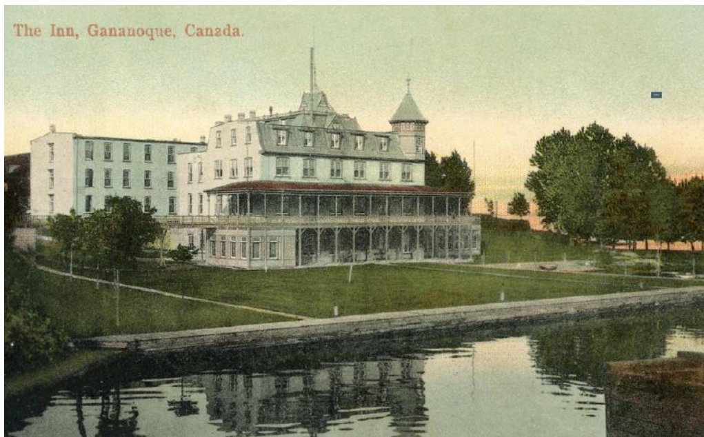
Gananoque Inn, ca. 1902, viewed from the northwest, following its adaptation as an inn. The current Inn is located to the rear of the mansard roof structure which had been adapted with water-facing verandas and corner tower. A tower was also added on the south elevation which gave greater St. Lawrence River waterfront attention (D. Rombough postcard and photographic collection).
