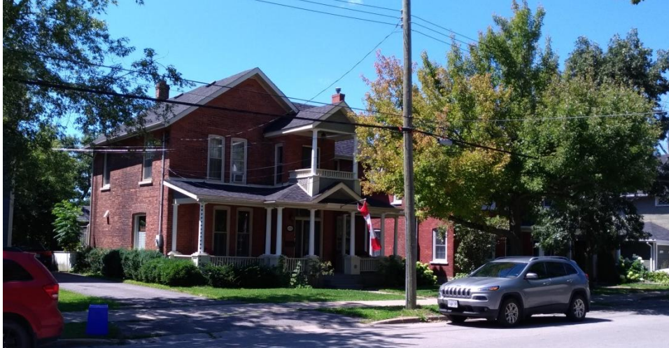
420 Stone Street South, viewed from the southeast (E. Tumak, Aug 2019).
