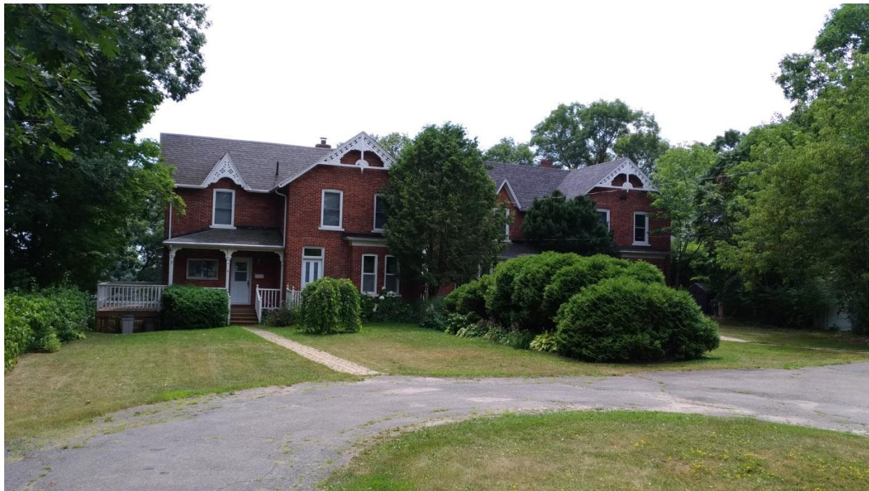
13 Windsor Drive, left, viewed from the northeast (E. Tumak, Aug. 2019).
