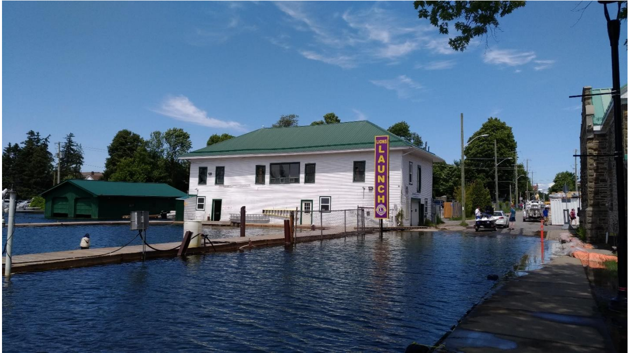
Water Street, Gananoque Boat Line Maintenance Facility, former Gananoque Yacht Club, later Blinkbonnie Boathouse, viewed from the southwest (E. Tumak, July 2019).
