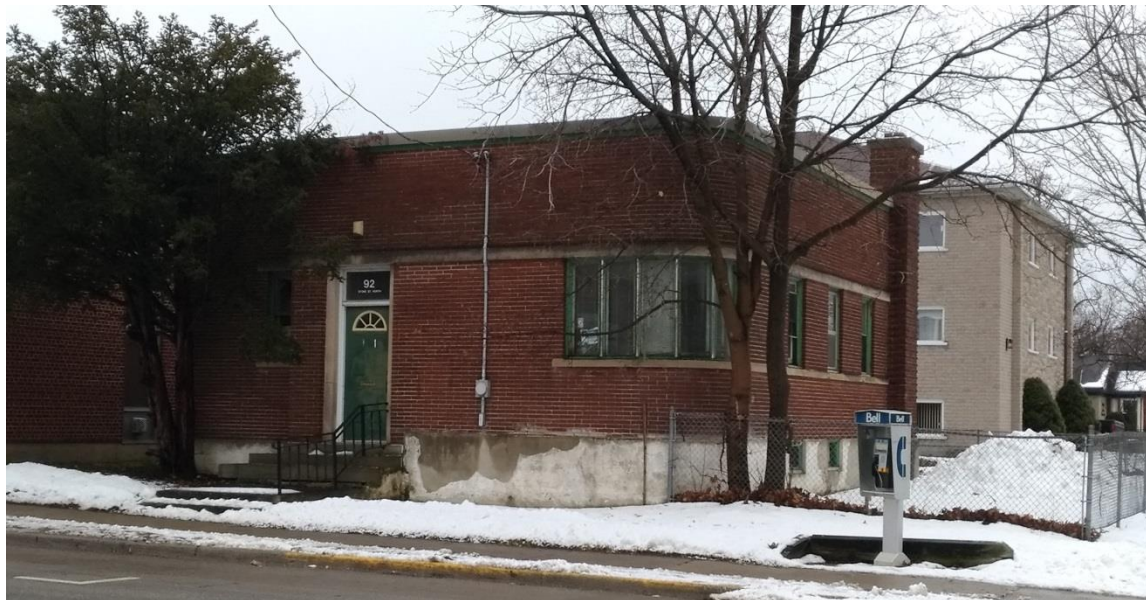
92 Stone Street North viewed from the northeast (E. Tumak, Jan. 2021).
