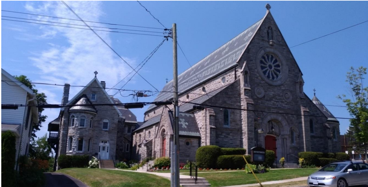
270 Stone Street South, St. John the Evangelist Rectory, left, viewed from the east (E. Tumak, July 2019).
