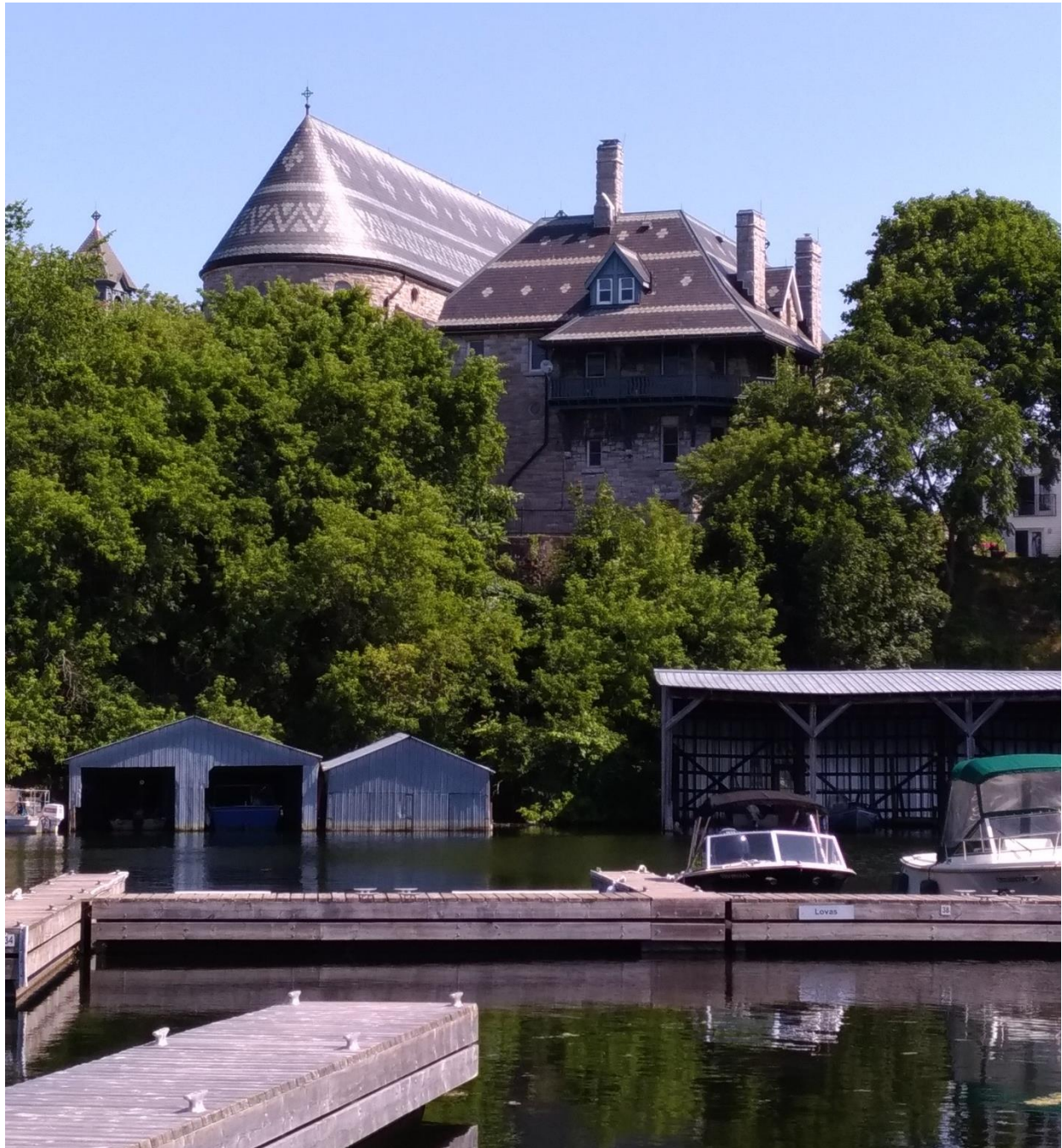
262 Stone Street South, St. John the Evangelist and St. Philomenas, and rectory (right/south) viewed from the west from the Gananoque River (E. Tumak, July 2019).
