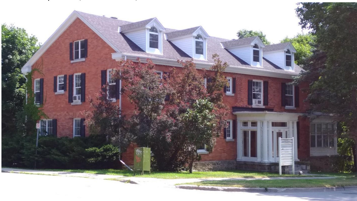
215 Stone Street South, viewed from the northwest (E. Tumak, July 2019).
