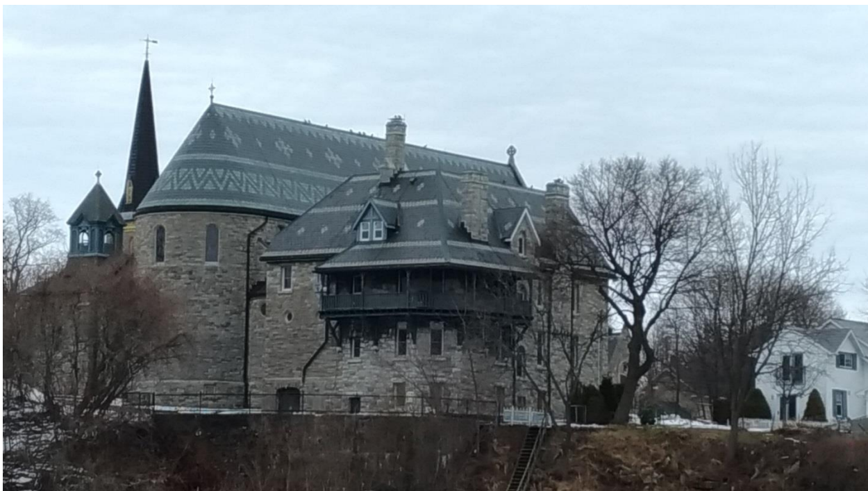
270 Stone Street South, St. John the Evangelist Rectory, right, viewed from the southwest (E. Tumak, January 2020).
