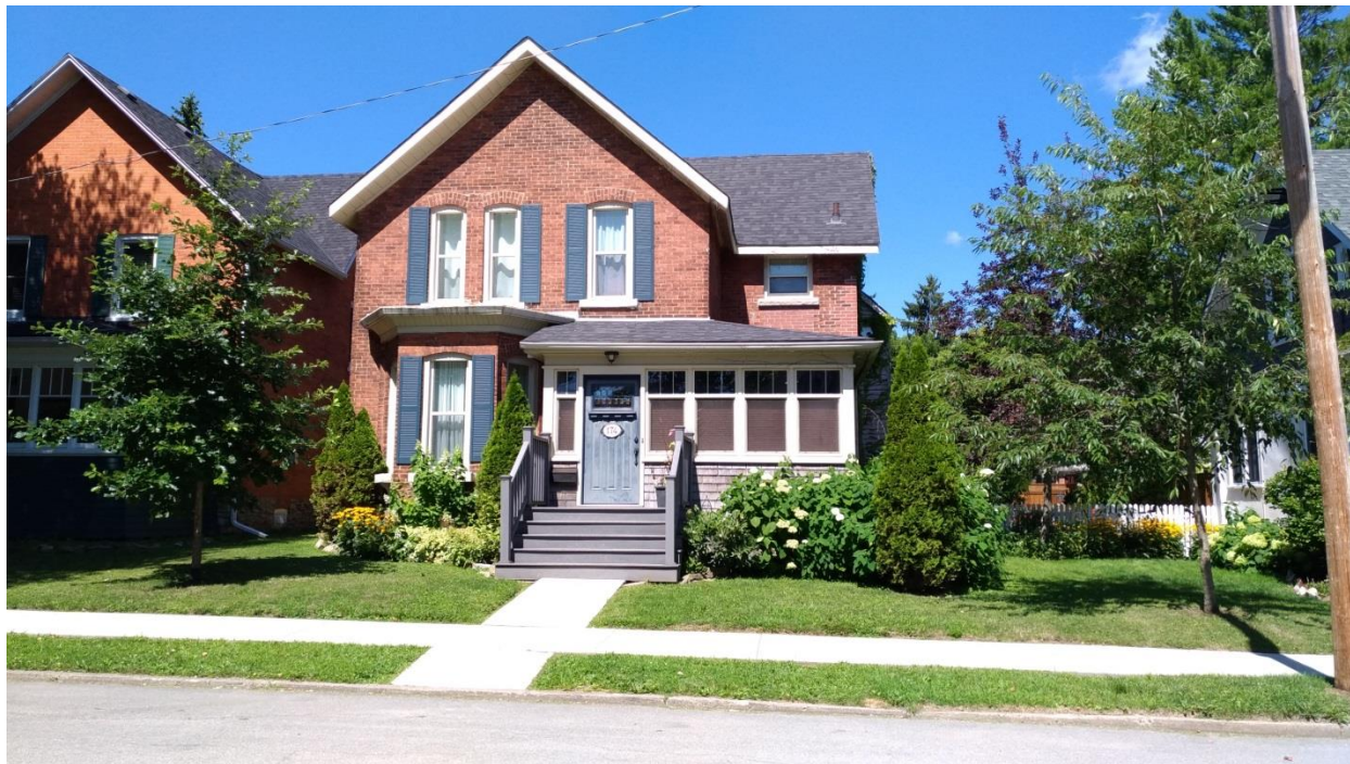
174 Sydenham Street, viewed from the south (E. Tumak, Aug. 2019).
