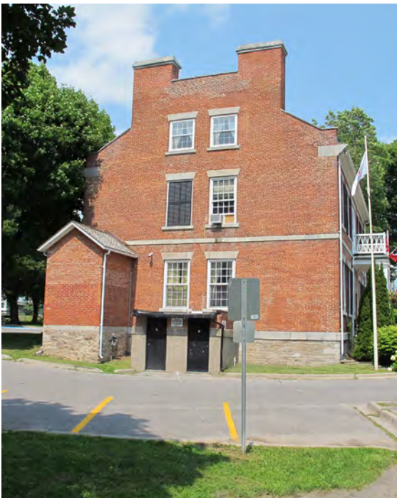
West elevation and existing additions
