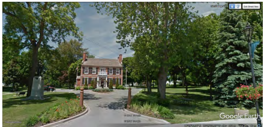
View from King Street of Town Hall and entrance landscape
