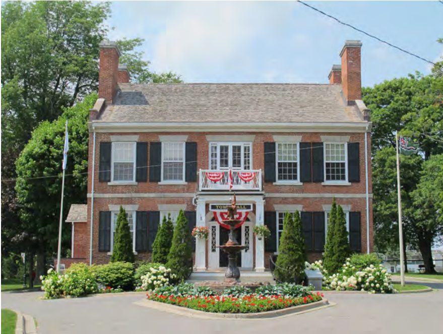
Main (south) elevation
