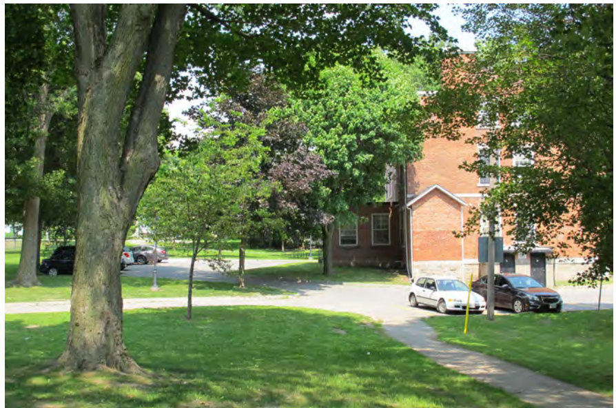
View E towards rear addition
