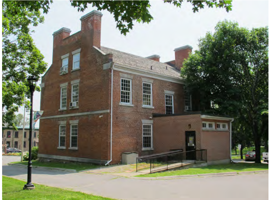
North and east elevations with rear addition
