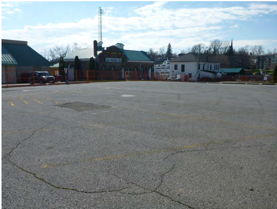
Image 14: Study area showing parking lot facing southwest.
