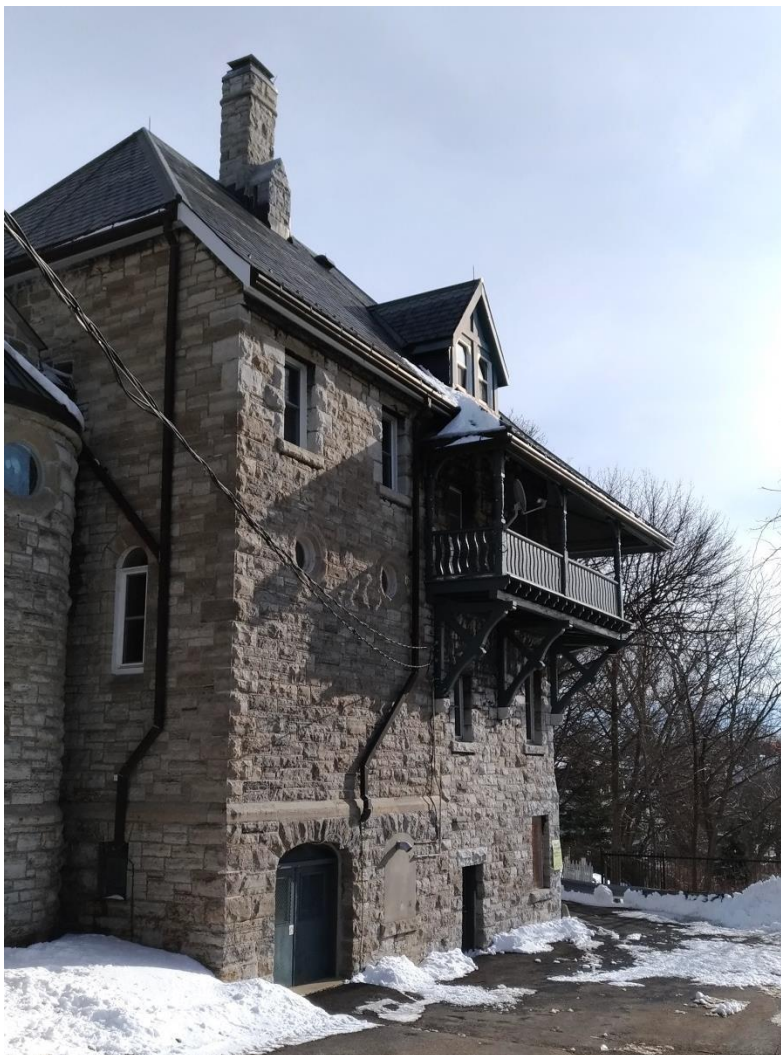
Figure 28: Rear/west elevation of the rectory (E. Tumak, Jan. 2020).
