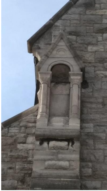
Figure 20: Detail of niche atop front façade buttress (E. Tumak, Jan. 2020).
