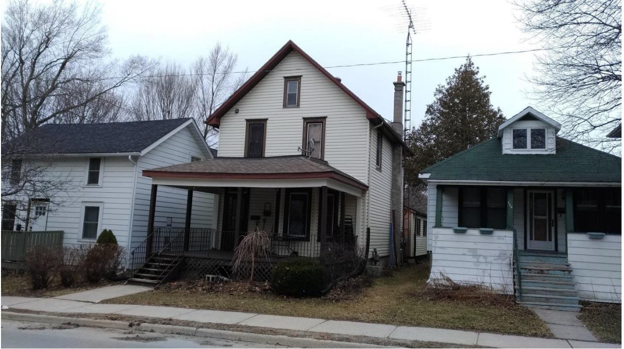
Figure 12: 132 North Street, Gananoque, former Delaney residence (E. Tumak, Feb. 2020).
