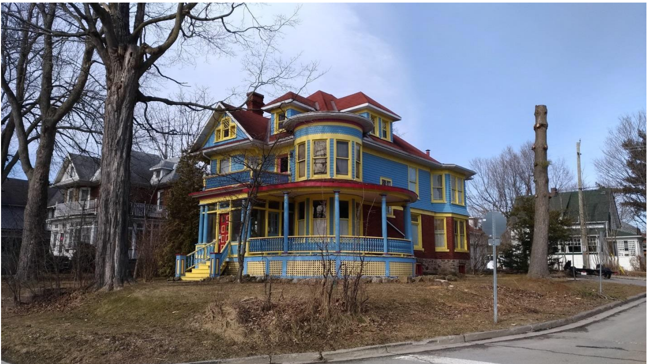
Figure 13: 198 South Street, viewed from the southeast, with colouration that was not present during the ownership of Eva Delaney, nor typical of its Queen Anne Revival style (E. Tumak, March 2020).
