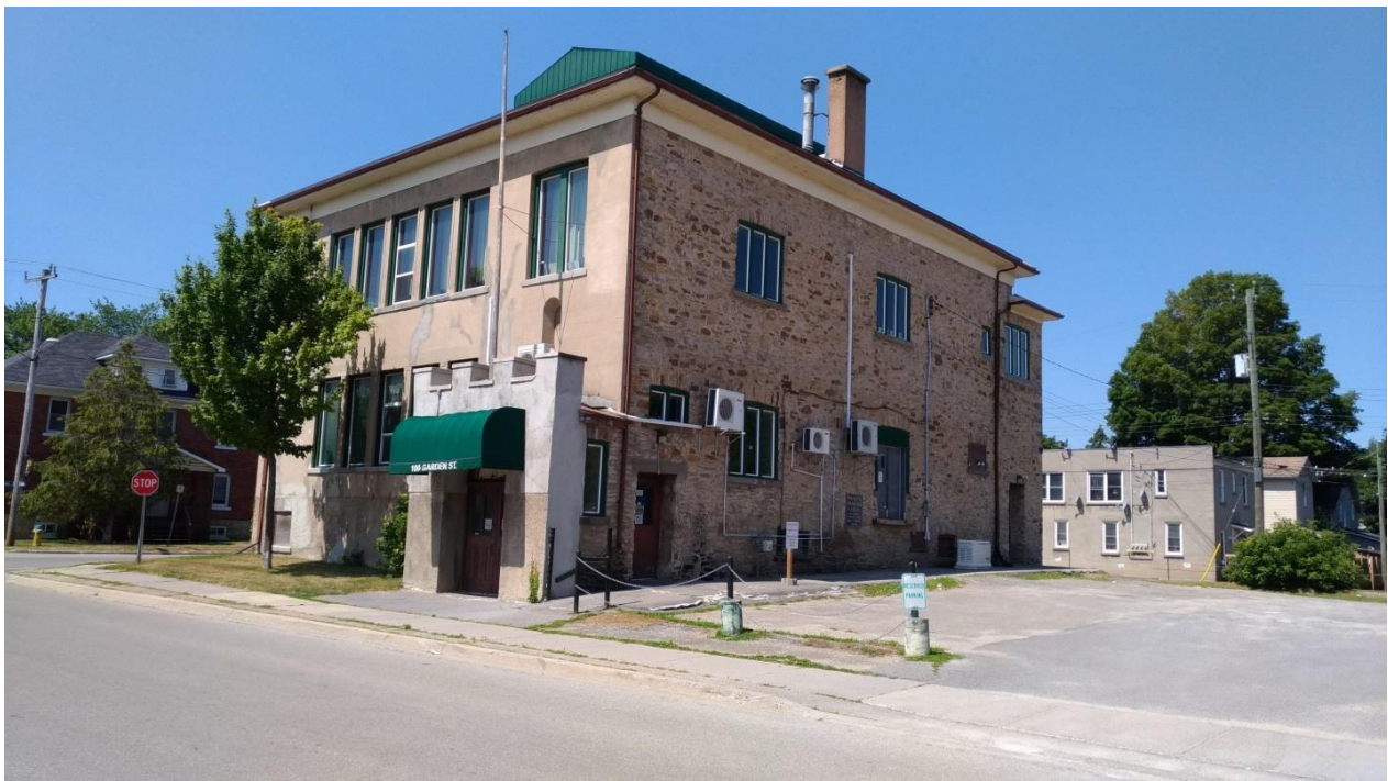
Figure 5: 100 Garden Street, viewed from the southeast (E. Tumak, July 2019).
