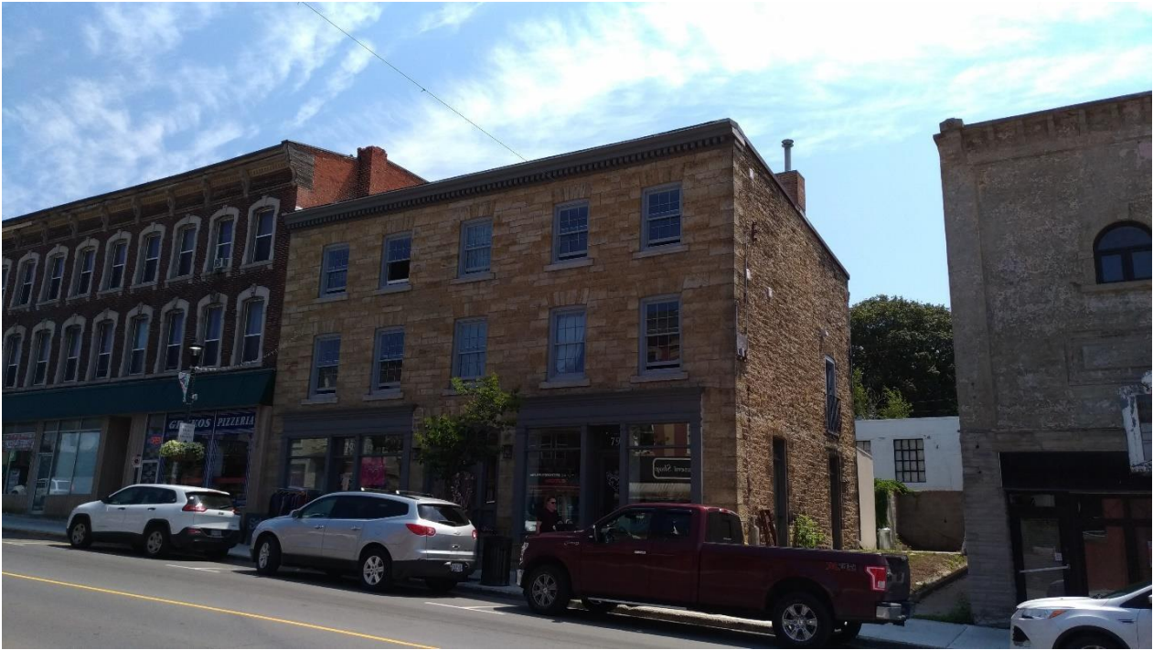
Figure 31: 79-81 King Street East, viewed from the northwest (E. Tumak, July 2019).
