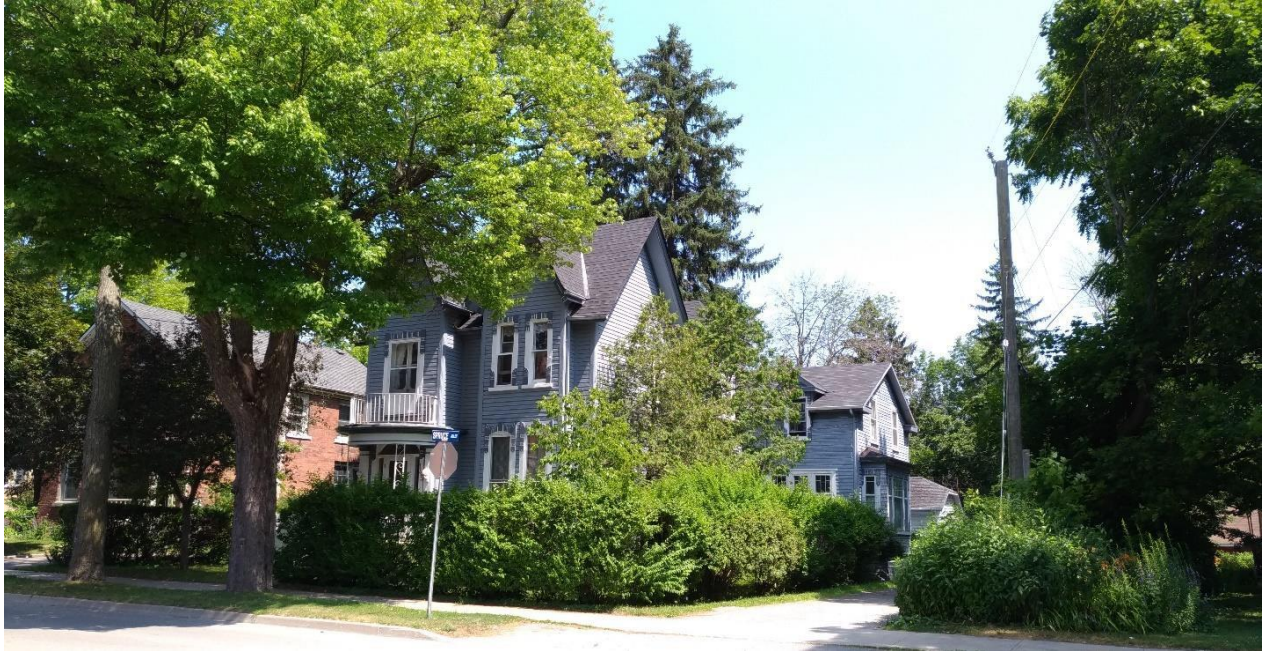
Figure 4: 145 Stone Street South, Gananoque, viewed from the southwest (E. Tumak, July 2019).
