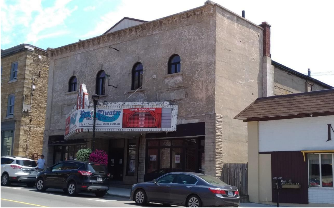
Figure 30: 75 King Street East viewed from the northwest (E. Tumak, July 2019).
