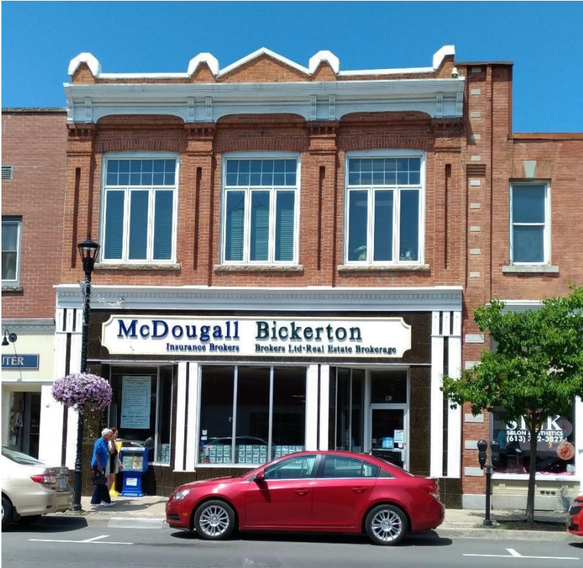
Figure 39: 170 King Street East, viewed from the south (E. Tumak, July 2019).
