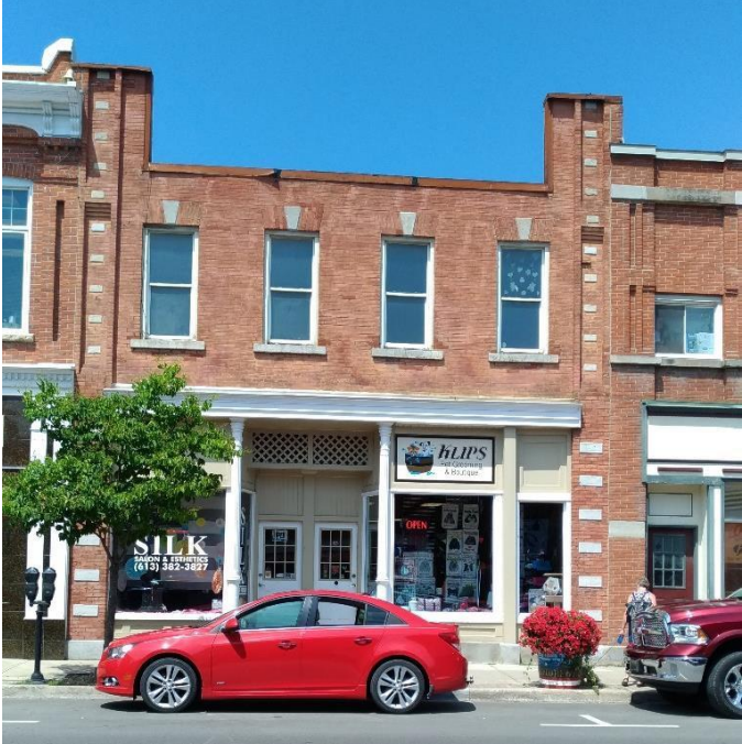
Figure 40: 176 King Street East, viewed from the south (E. Tumak, July 2019).
