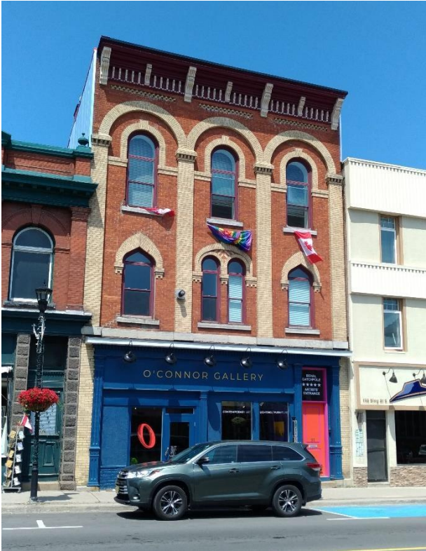
Figure 37: 130 King Street East, viewed from the south (E. Tumak, July 2019).
