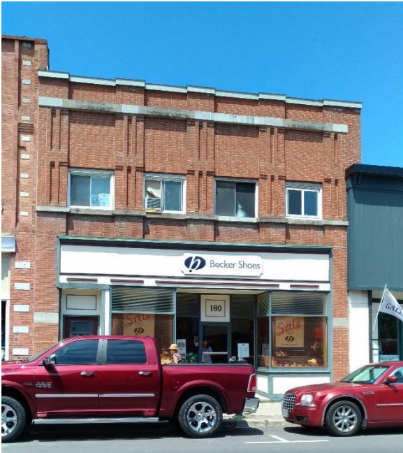
Figure 41: 180 King Street East, viewed from the south (E. Tumak, July 2019).
