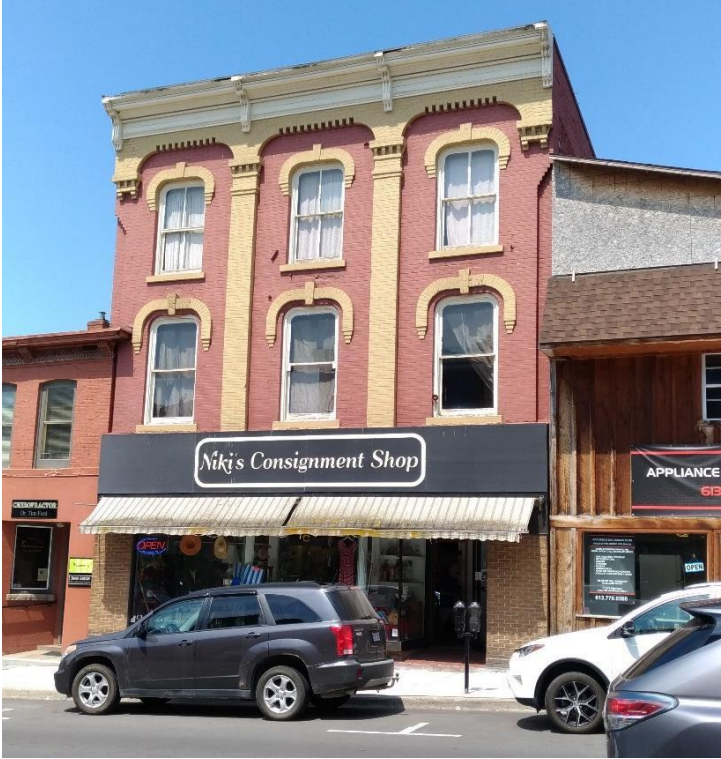
Figure 32: 84 King Street East, viewed from the south (E. Tumak, July 2019).
