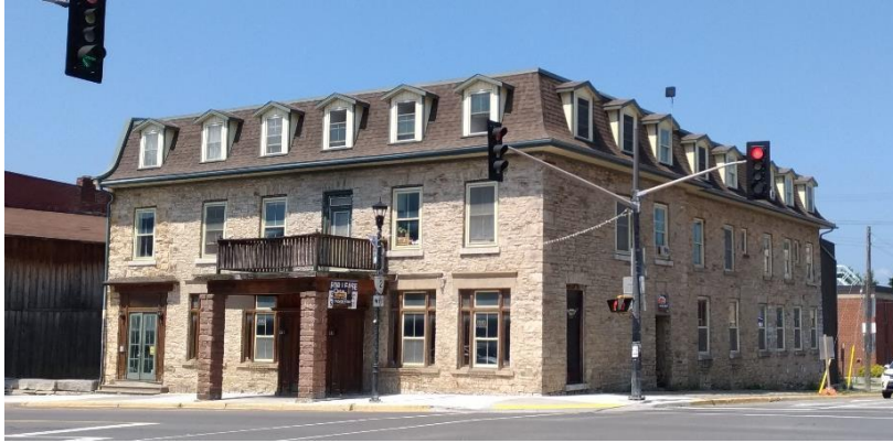
Figure 34: 98 King Street East, ca. 1885, refurbished 2003-04 after serious fire damage, former Cheever's House and Provincial Hotel (designated Pt. IV, by-law 2005-63), viewed from the southeast (E. Tumak, July 2019).
