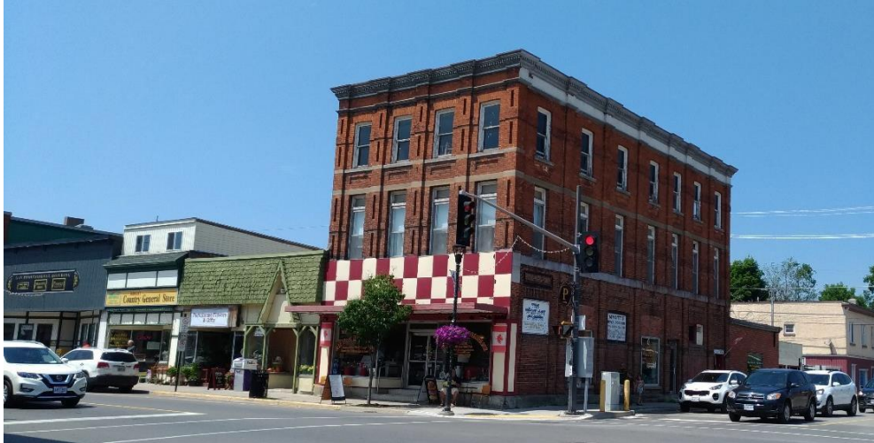
Figure 42: 198 King Street East, viewed from the southeast (E. Tumak, July 2019).
