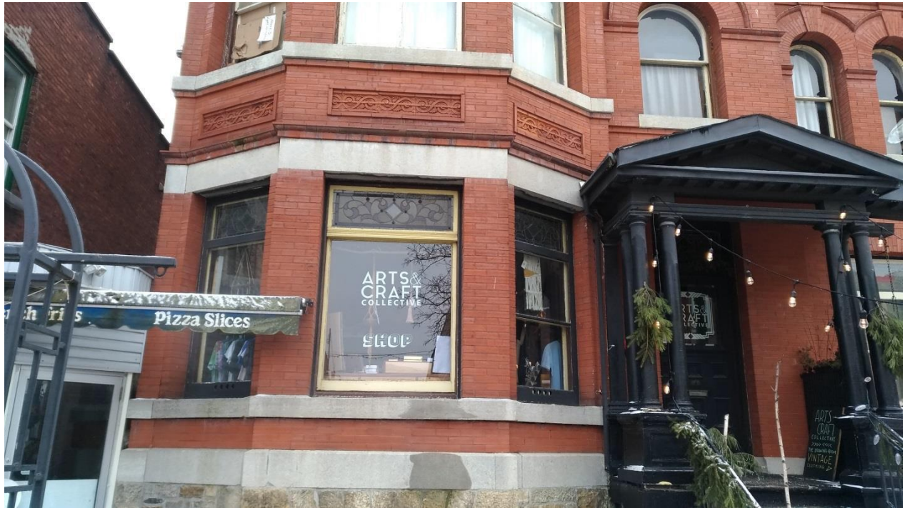
Figure 17: Showing the lower level of the front window bay with the scroll pattern of the terra cotta panels between the ground and second levels (E. Tumak, Jan. 2020).
