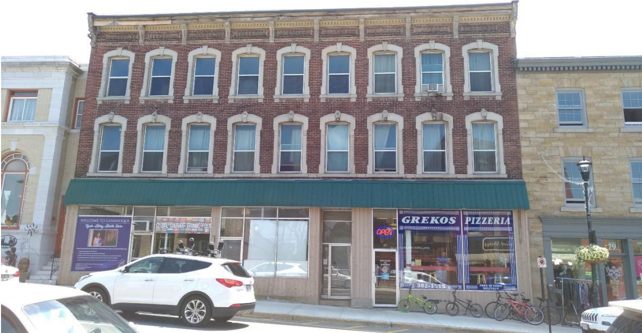
Figure 33: 79-87 King Street East (E. Tumak, July 2019).
