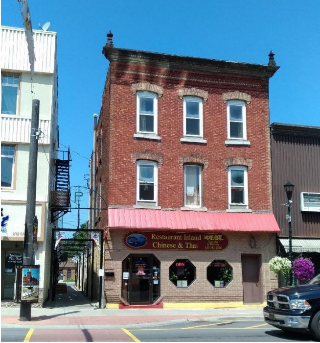
Figure 38: 146 King Street East, viewed from the south (E. Tumak, July 2019).
