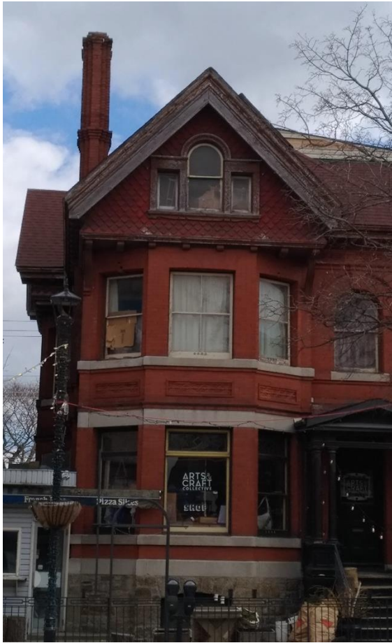
Figure 16 - left: Two-storey bay window topped by a Palladian window under a gable with shingle surround (E. Tumak, March 2020).
