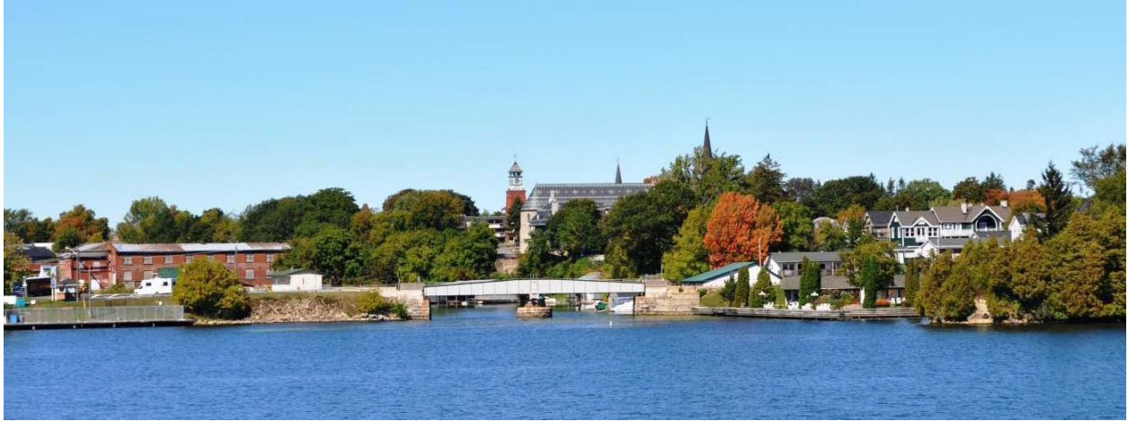
Figure 40: Panoramic view from the St. Lawrence River looking north to the Gananoque River, showing from left to right, the Brick Building of 185 Mill Street, the Swing Bridge crossing the Gananoque River, the brick Clock Tower, the stone St. John the Evangelist Roman Catholic Church, and the spire of St. Andrew's Presbyterian Church (photo J. McKendry, March 2014, in "185 Mill Street and 15 Clarence Street" Heritage Impact Statement, Appendix A, cover page).
