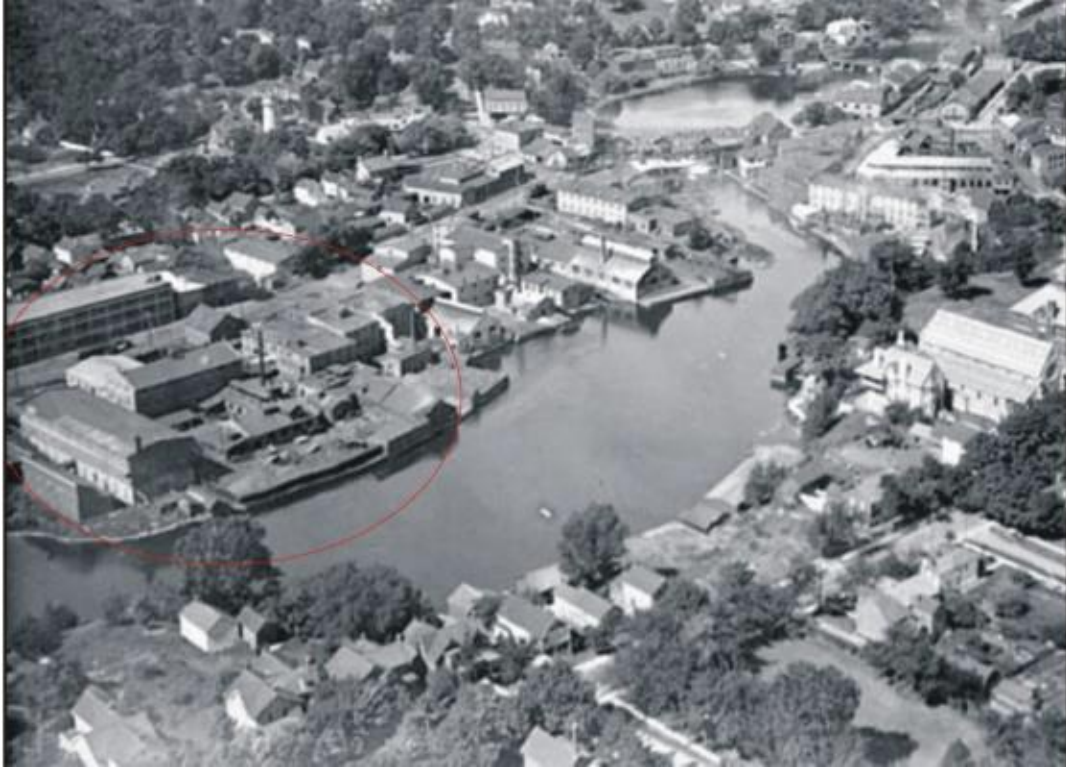
Figure 29: Aerial view from the southeast, 1920, showing 185 Mill Street in the lower left circled in red. The Brick Building is in the far left centre and the Stone Building to its immediate right/north, with the three-storey former Parmenter & Bulloch/Textron Building immediately to the west/left. In this image there are structures to the immediate east/right, north, and west/left of both the Stone and Brick Buildings (LAC, PA-30656).
