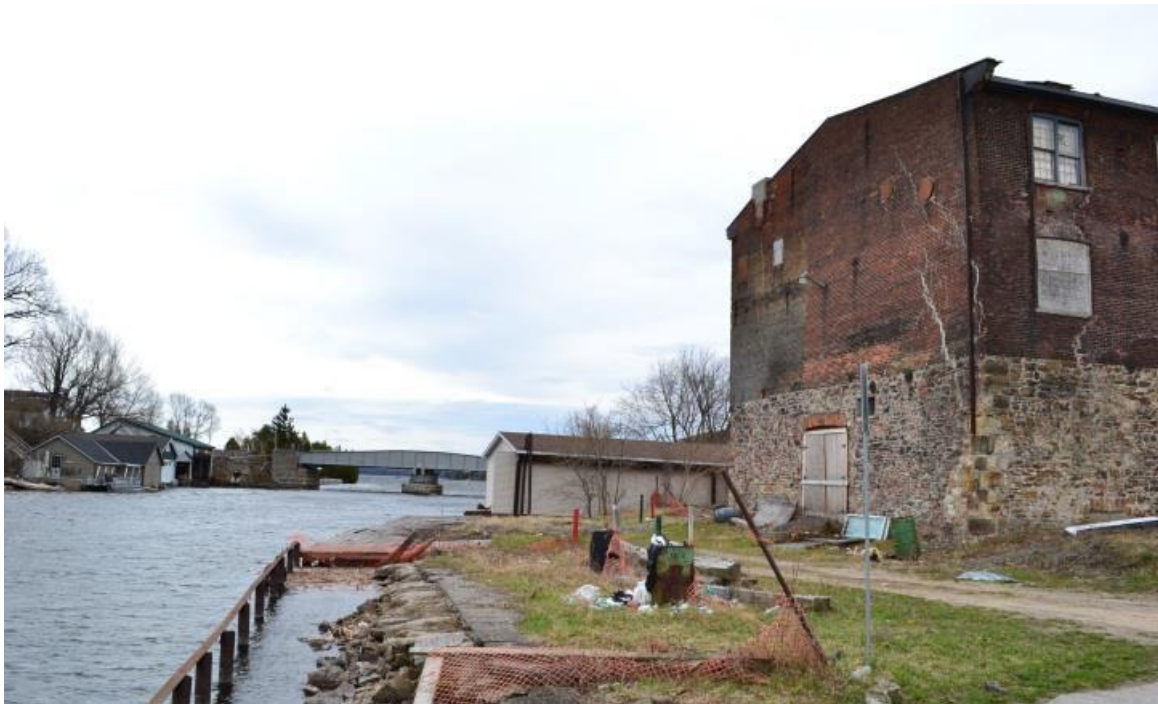
Figure 11: Brick Building, 185 Mill Street, waterfront/east elevation, showing the caps for interior metal tie rods between the main and upper levels on the west/left and north/right elevations (source, Peer Review: Heritage Impact Assessment, 2014, p. 3.)
