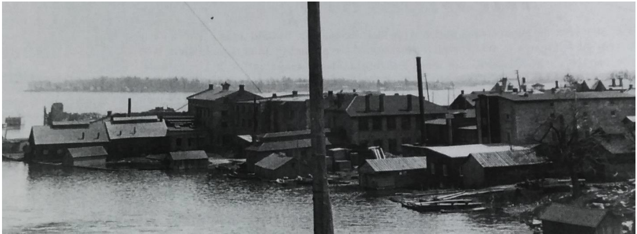
Figure 17: View of the Stone Building, 185 Mill Street, with its two end chimneys and small central ventilation cupola, seen to the left of the pole in the centre of the image. The Brick Building, which would be located perpendicular to the left, is not present due to almost complete fire damage (save for the foundations which are partially visible) in ca. 1892 (Gananoque Historical Society Newsletter, Sept. 2013, no. 60, p. 1639).
