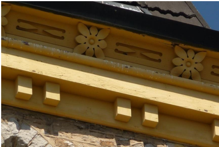
Figures 10-12: top – St. Andrew's, wood cornice detail showing decorative classical and floral motifs; middle – weather vane topping the spire; and bottom – concave eave ornamenting the church (photos: E. Tumak, May 2015).
