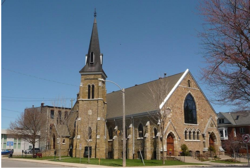
Figure 22: Grace United Church (former Methodist Church), viewed from the southwest (photo: E. Tumak, May 2015).
