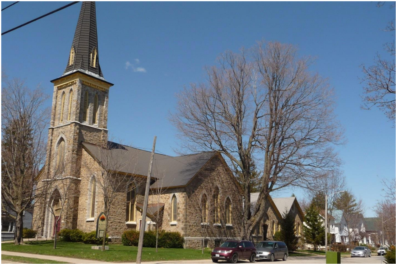
Figure 2: St. Andrew's Presbyterian Church, Gananoque, viewed from the southwest, with the sanctuary on the west/left and the Gracey Hall on the east/right (photos E. Tumak, May. 2015).
