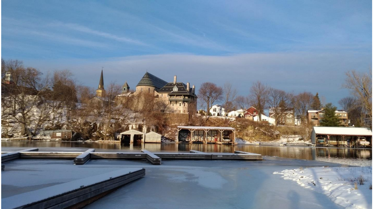
Figure 35: 270 Stone Street South, viewed from the southwest (E. Tumak, January 2020).
