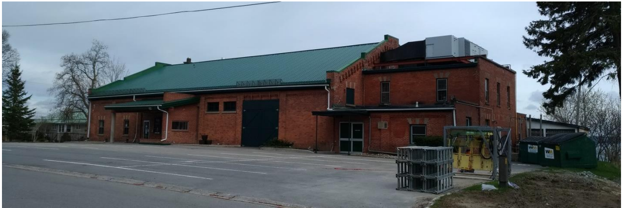
Figure: 1000 Islands Playhouse (former Drill Hall, then Firehall and Police Station), 185 South Street, viewed from the northwest, showing a later addition to the right/west (E. Tumak, May 2020).
