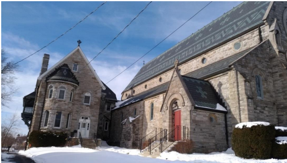
Figure 21: South side of St. John's, showing from right to left, the south entrance, the outward extending confessional, the link between the church and the rectory, and the rectory (E. Tumak, Jan. 2020).
