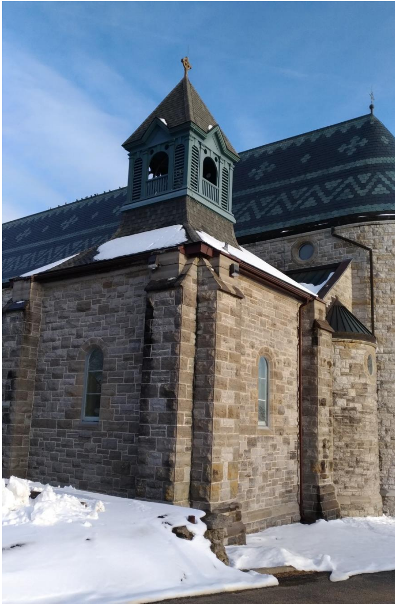
Figure 26: 'Tower' supporting the belfry (E. Tumak, Jan. 2020).
