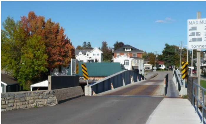
Figures 7-9: left – Current bridge deck showing the steel grate deck of the vehicle lane on the left and the pedestrian walk on the right, viewed from the west (photo E. Tumak, Sept. 2013); middle – Prince of Wales Drive/Hogs Back Swing Bridge, Rideau Canal System, Ottawa, showing the asymmetrical structure swinging from one end only, and partially open (Wikimedia Commons, July 2006.; and bottom – Little Current Swing Bridge, Northeastern Manitoulin and the Island, Ontario (Wikipedia).
