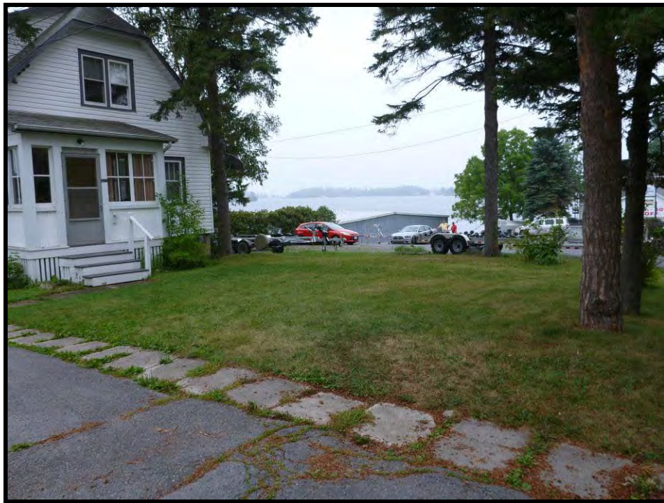
Figure 23. View of the dwelling at 161 South Street, looking southwest. (PR13-24D03)
