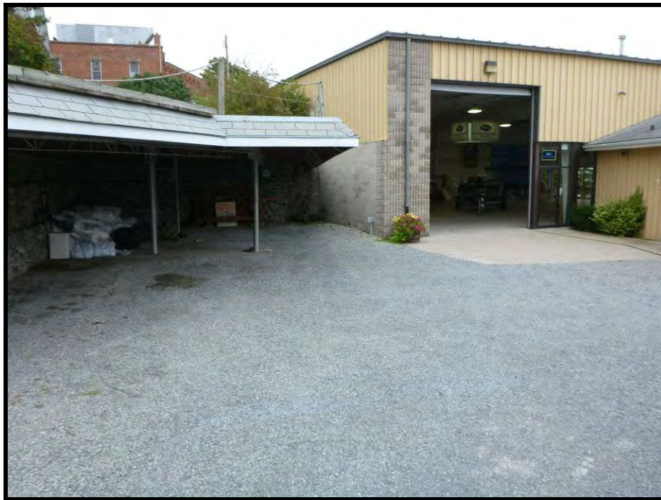
Figure 25. View of the storage area and rear of the marina showroom, looking east. (PR13-24D06)
