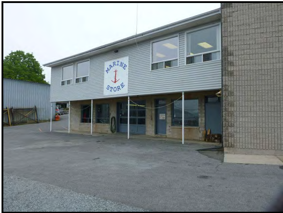
Figure 27. View of the Marine Store building, looking northwest. (PR13-24D12)
