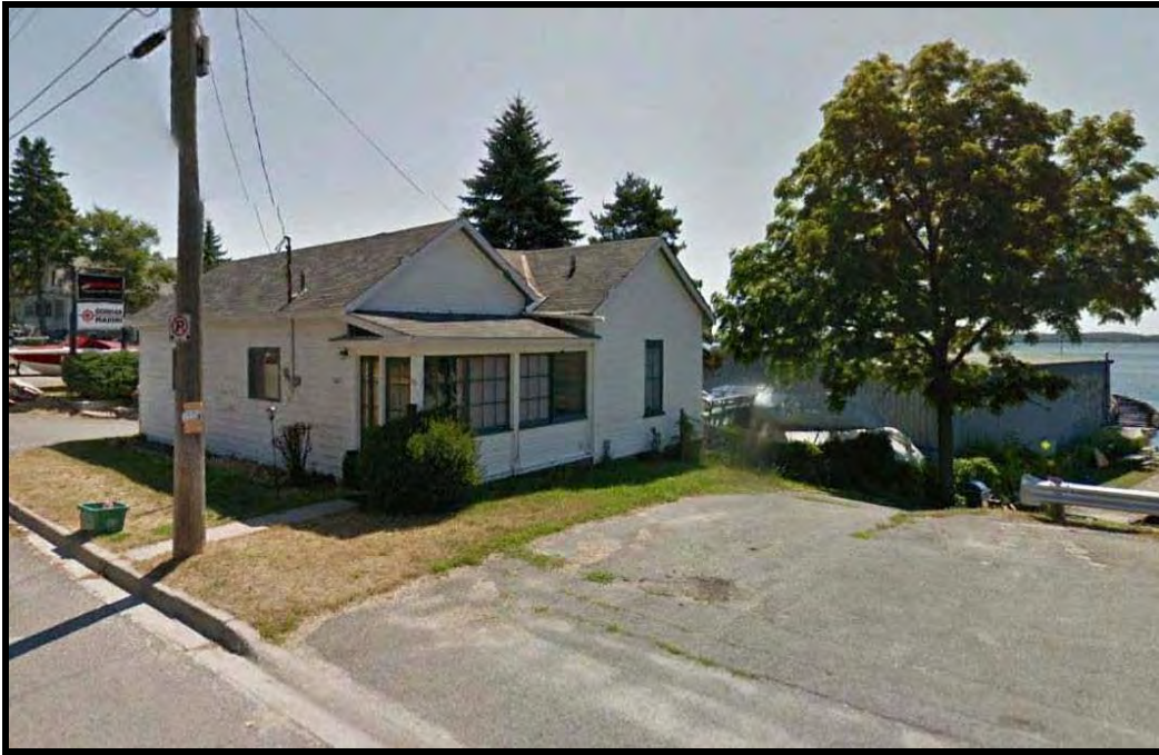
Figure 21. View of the dwelling at 119 South Street, looking southeast. (PR13-24D18)
