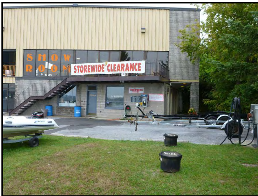
Figure 26. View of the main marina building, looking north. (PR13-24D11)
