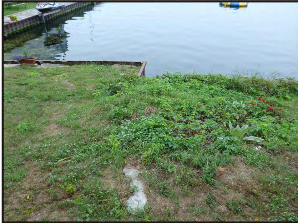
Figure 31. Foundation for old boathouse, looking south. (PR13-D22)
