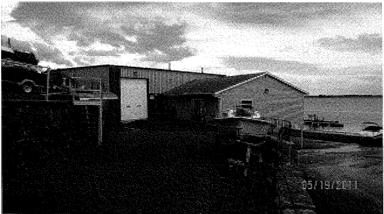
Photo 2 – Easterly view of main building.
