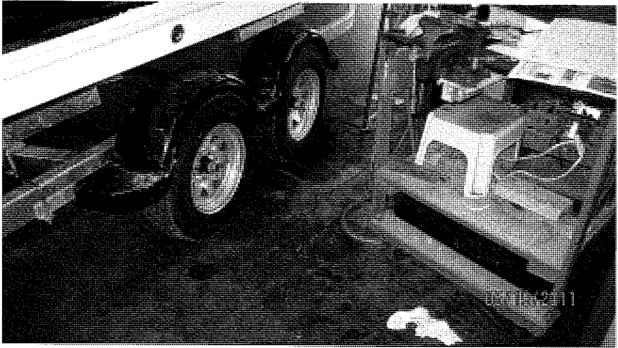
Photo 19 – Floor drain in the maintenance shop. Reportedly, the floor drain is pumped to the sanitary sewage drain.
