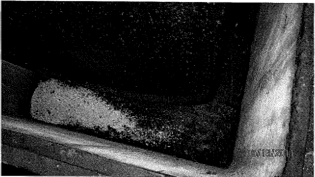
Photo 22 – View of staining inside the concrete secondary containment.
