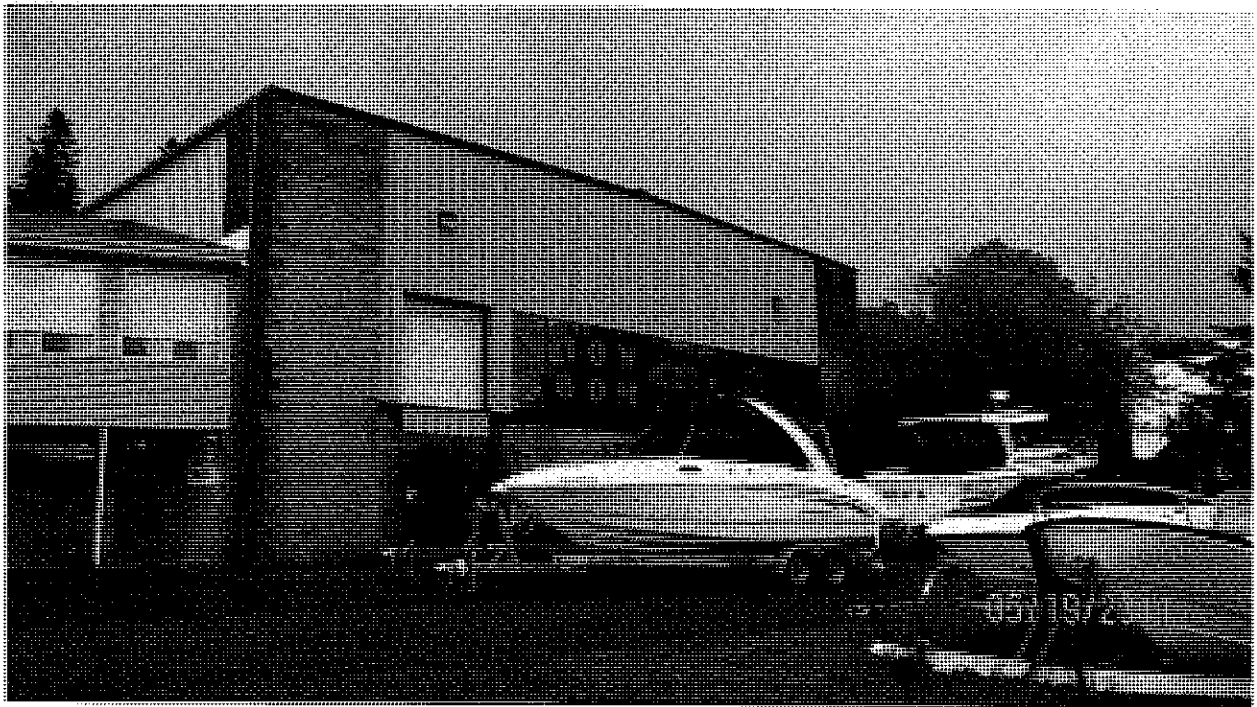
Photo 4 – Northerly view of show room in the main building.
