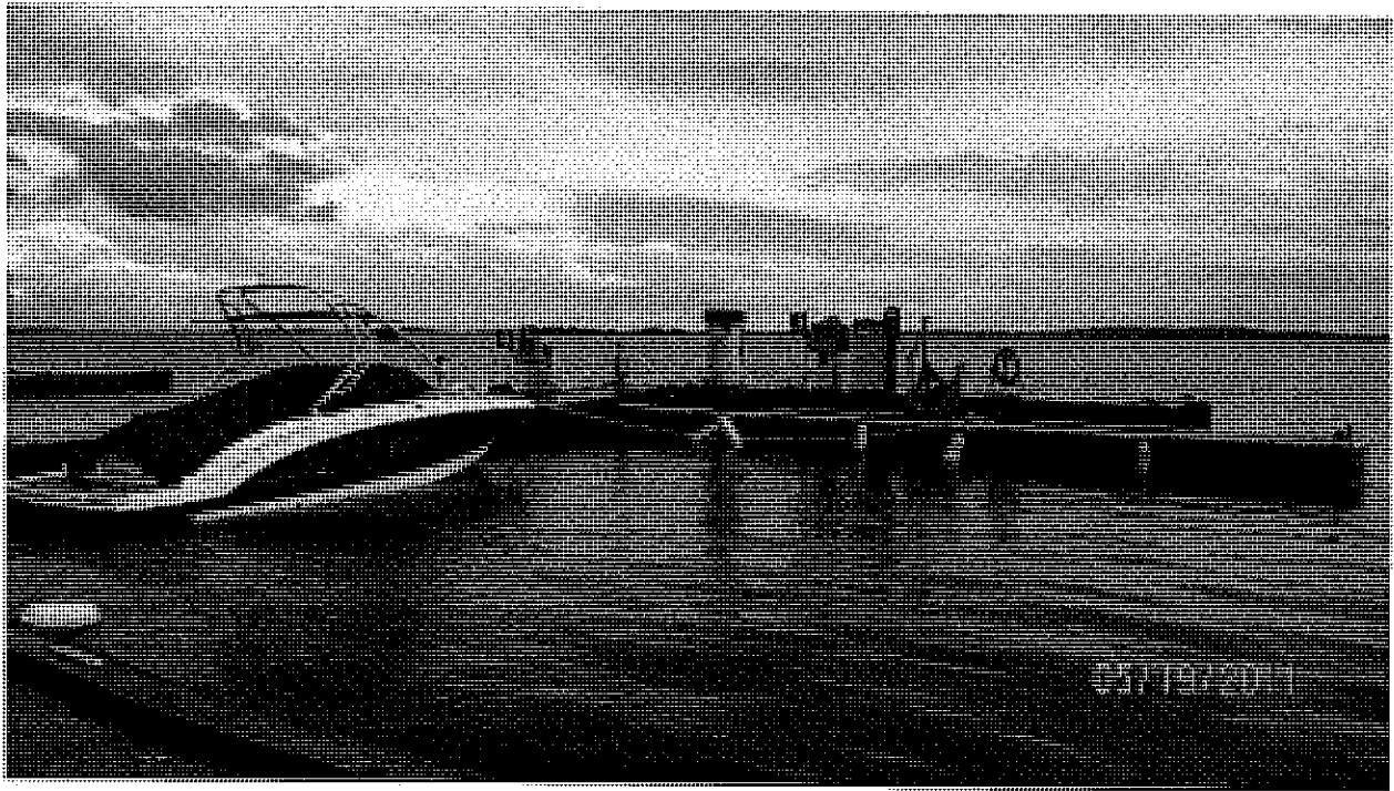
Photo 9 – View of fuel pump island.
