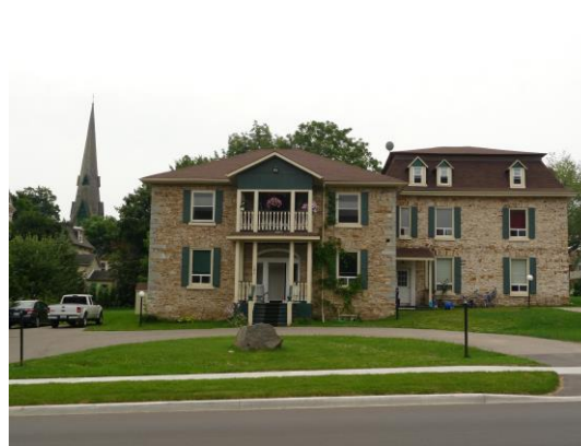
Figures 24 – 25: left – Beaver Hall Bed and Breakfast, 75 King St. W., Gananoque (photo E. Tumak, Jan. 2008); right – 181 King St. W., Gananoque—the wing at the right/west is a later addition (photo E. Tumak, July 2009). Note both are constructed of sandstone.
