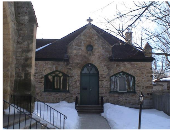
Figures 16 – 17: left – 1 st Christ Church rectory, 40 Princess St., viewed from the northeast, built after the first phase of the church, enlarged at rear, late 1910s (photo E. Tumak, July 2009); right – Christ Church Parish Hall, east/Church St. elevation (photo E. Tumak, Jan., 2008).
