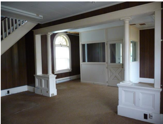
Figure 13: left – Gananoque Pump House, ground level interior of the engineer's residential accommodation, constructed 1925-26, looking towards the exterior entrance (photo E. Tumak, July 2009).
