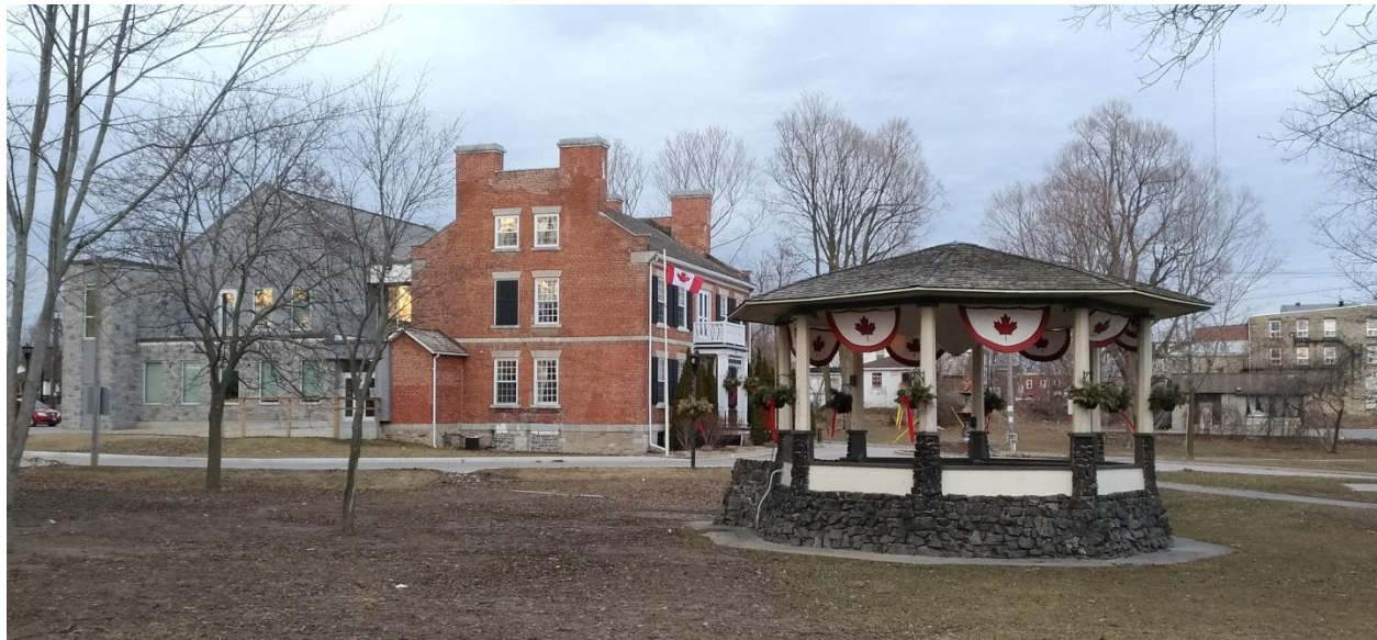
Figure 1: Gananoque Bandshell, 30 King Street East, viewed from the west, with Town Hall in the background (E. Tumak, March 2020).
