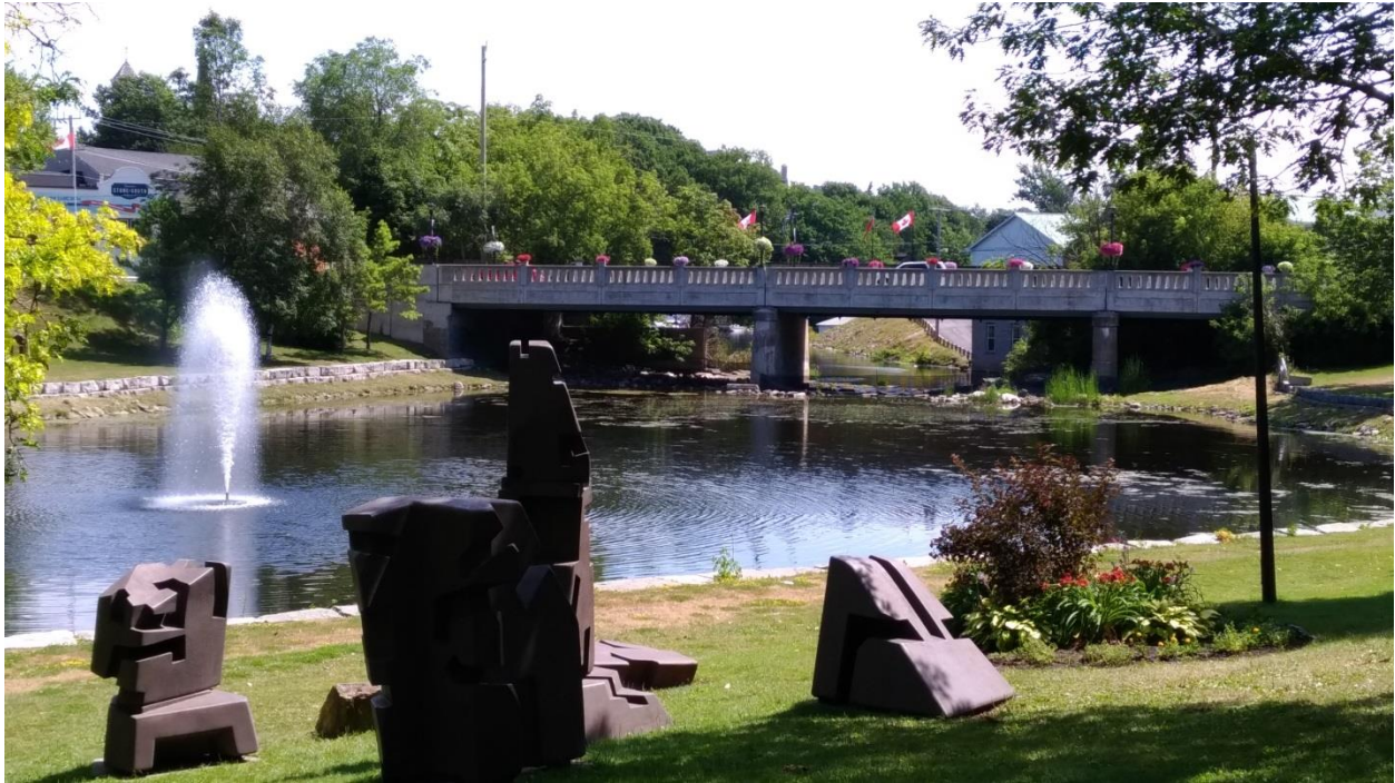
Figure 19: King Street Bridge, viewed from the northwest (E. Tumak, July 2019).
