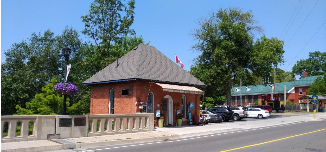
Figure 17: 2 King Street East, viewed from the southwest with the north side of the King Street Bridge (E. Tumak, July 2019).
