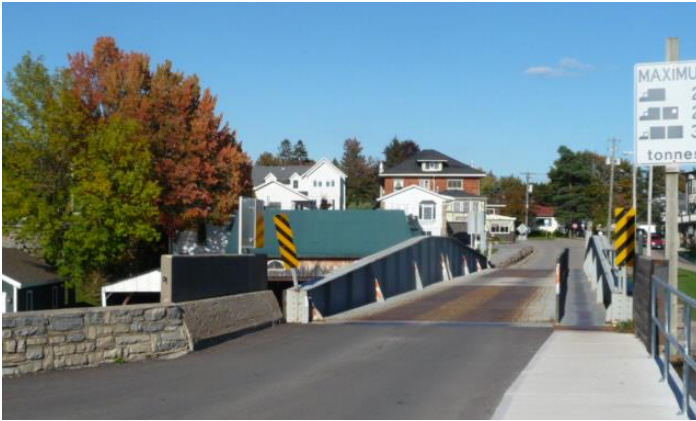
Figures 7-9: left – Current bridge deck showing the steel grate deck of the vehicle lane on the left and the pedestrian walk on the right, viewed from the west (photo E. Tumak, Sept. 2013); middle – Prince of Wales Drive/Hogs Back Swing Bridge, Rideau Canal System, Ottawa, showing the asymmetrical structure swinging from one end only, and partially open (Wikimedia Commons, July 2006.; and bottom – Little Current Swing Bridge, Northeastern Manitoulin and the Island, Ontario (Wikipedia).
