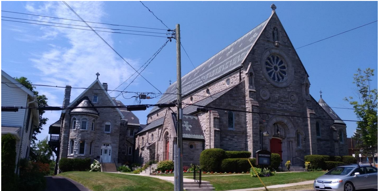
Fig. 2 Front Elevation (Façade) [source: E. Tumak, July 2019]
