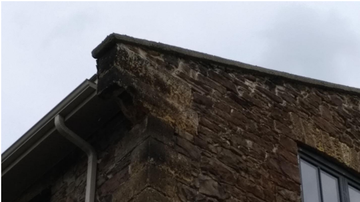
Fig. 7: Detail showing stone corbel treatment [source: E. Tumak, July 2020].
