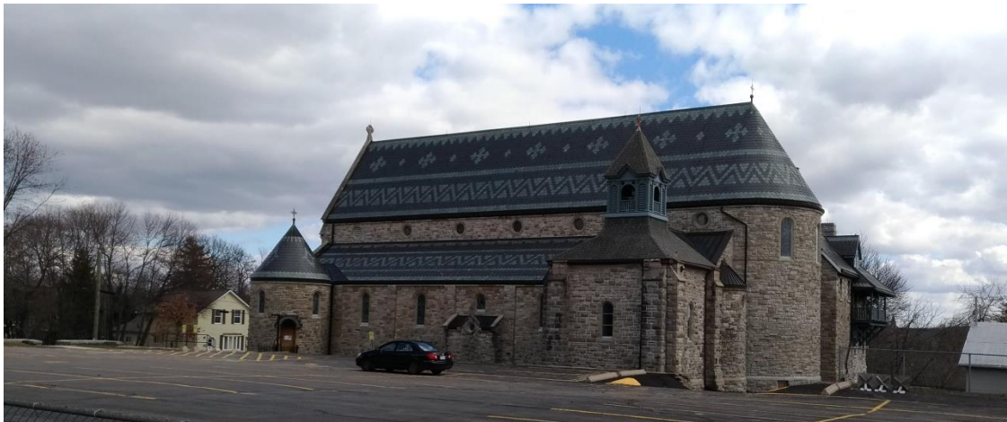
Fig. 1: North elevation, particularly fine patterned dichromatic slating. [source: E. Tumak, March 2020]
