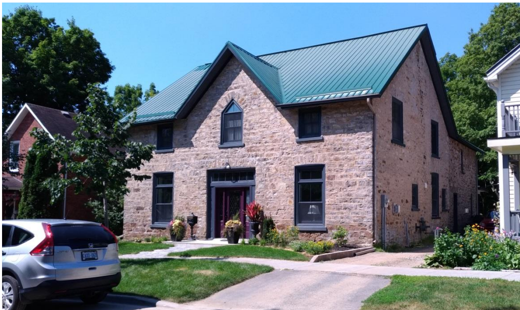
Figure 7: 40 Princess St., the first Christ Church Rectory, viewed from the northeast, built after the first phase of Christ Church 1857-58, enlarged at the rear late 1910s (photo E. Tumak, July 2009).
