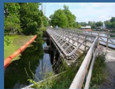
Pedestrian Bridge over Gananoque River
