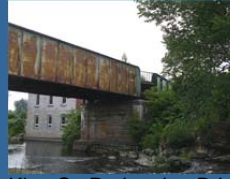
King St. Pedestrian Bridge
