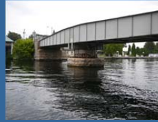
Water Street Swing Bridge
