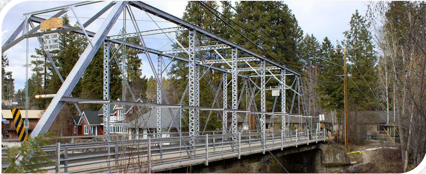
'Single Lane Truss – Bridge Street,' Town of Bigfork, Montana, bigfork.com
