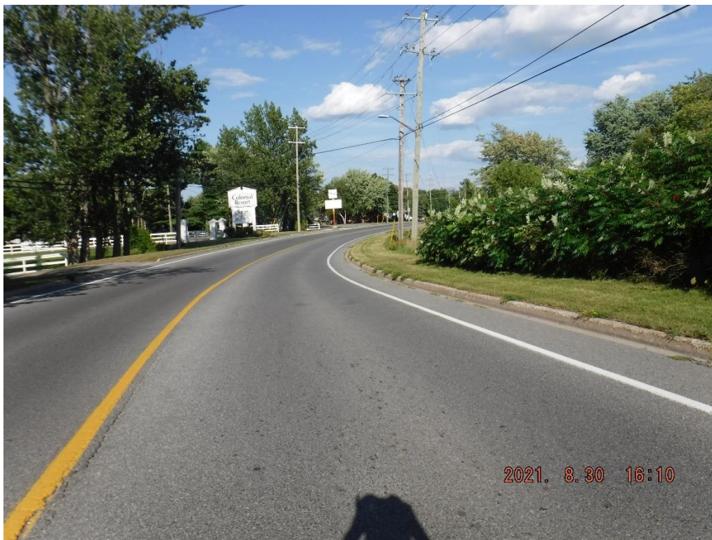
Photo 1: View of driveway for westbound vehicles entering the Town (vegetation within right-of-way to be removed) where the driveway is to be located beyond the vegetated right-of-way
