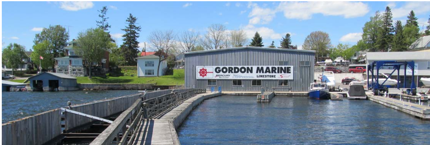
Figure 2.5 : Western Portion of Existing Shoreline
