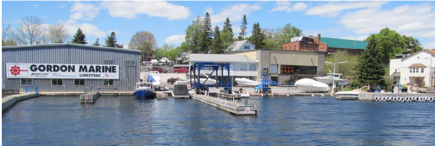
Figure 2.5: Eastern portion of Existing Shoreline
